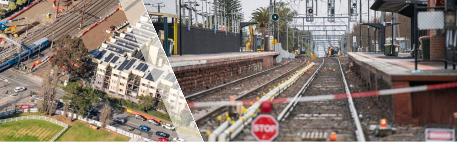
Glenhuntly Station during recent works
