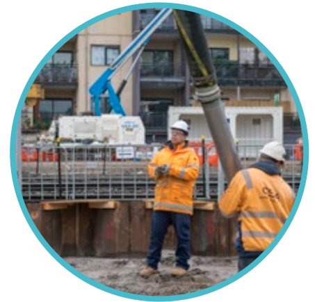
Piling works continue in Glen Huntly
