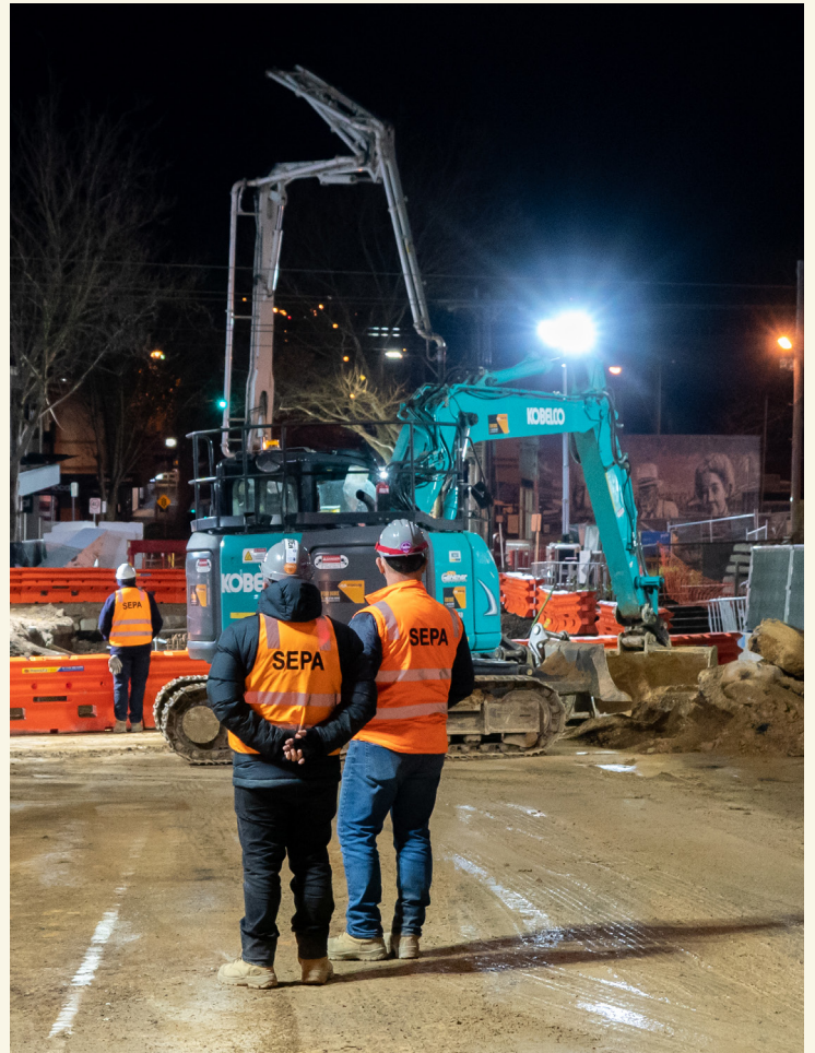
Night works to install beams under Union Road.
