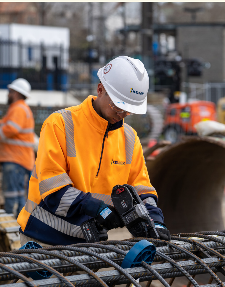
Preparing the steel reinforcing for piles.
