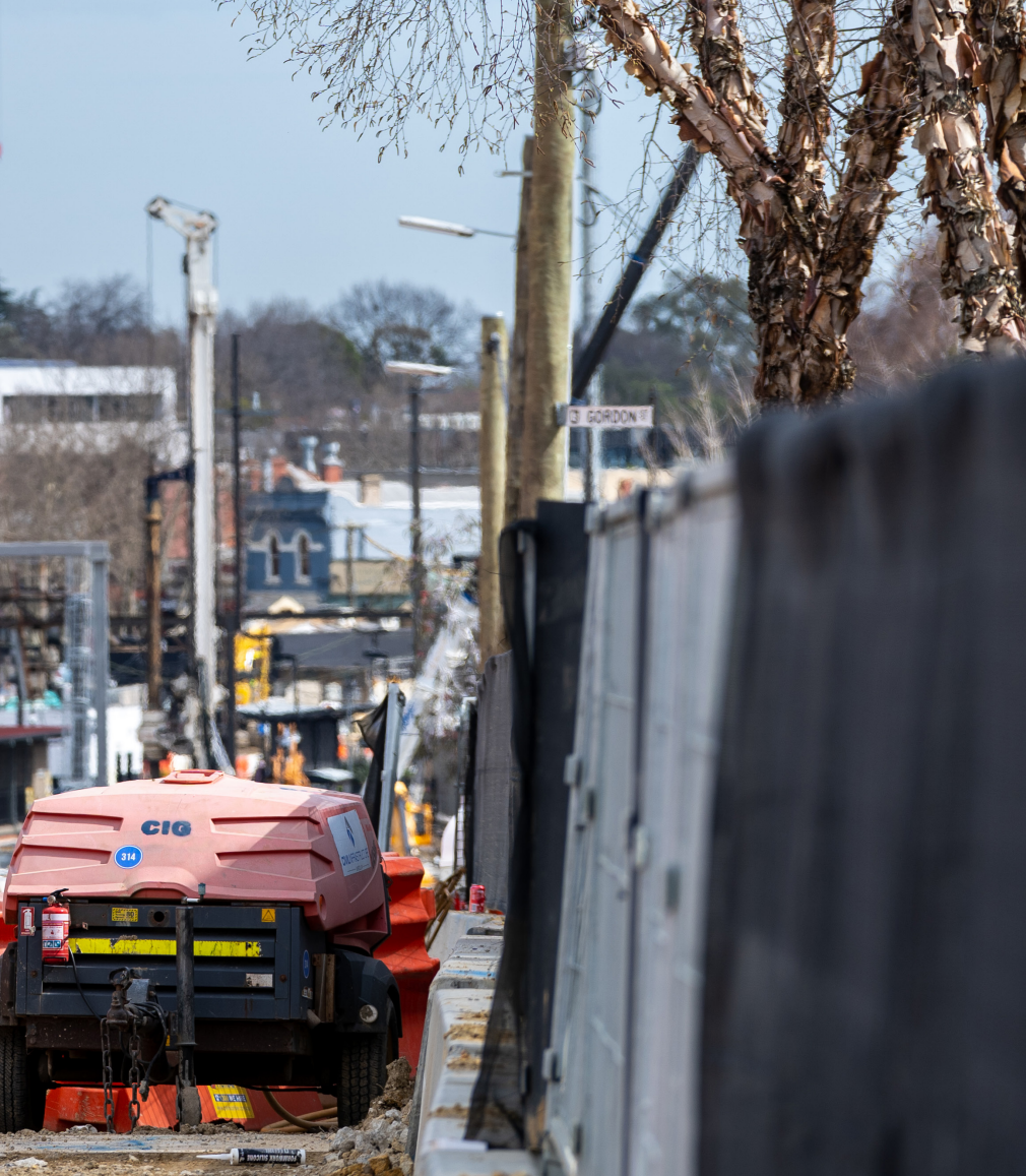
Works in Beresford Street.
