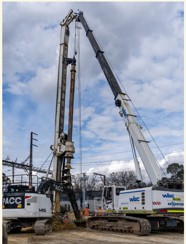
Piling works along the rail corridor.
