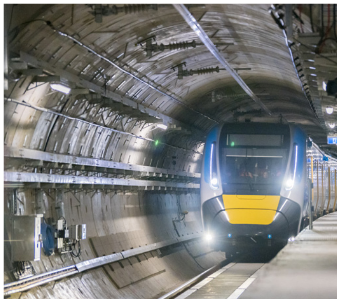
The first test train entering the Metro Tunnel, July 2023
