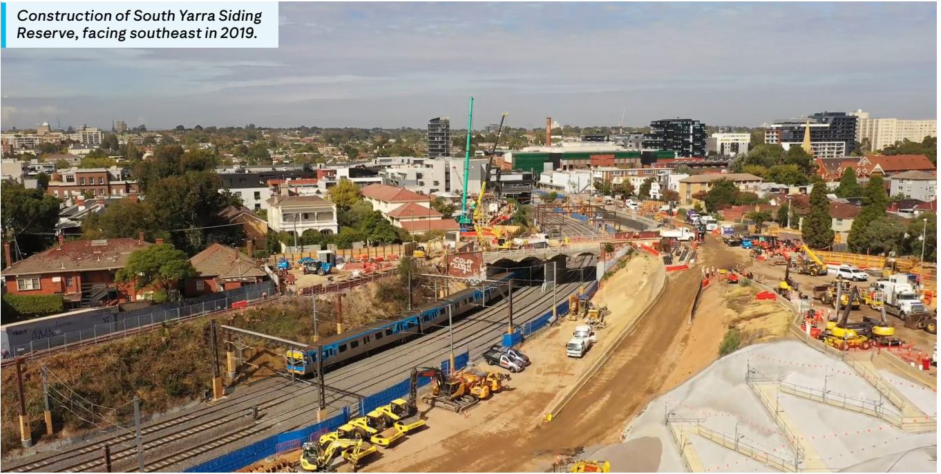
Construction of South Yarra Siding Reserve, facing Melbourne CBD in 2019.
