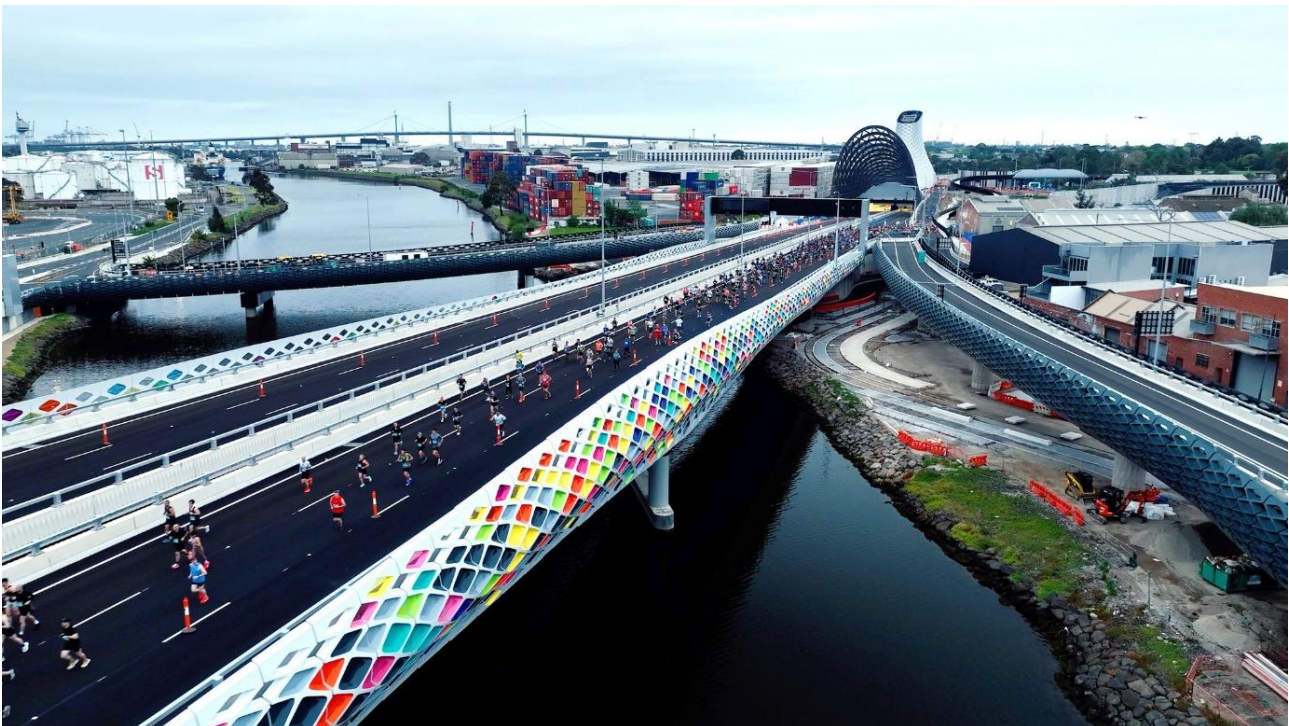
Photo 2 – Elevated roadway across the Maribyrnong River on Project opening day (Source: WGTP VIDA Roads, November 2025)
