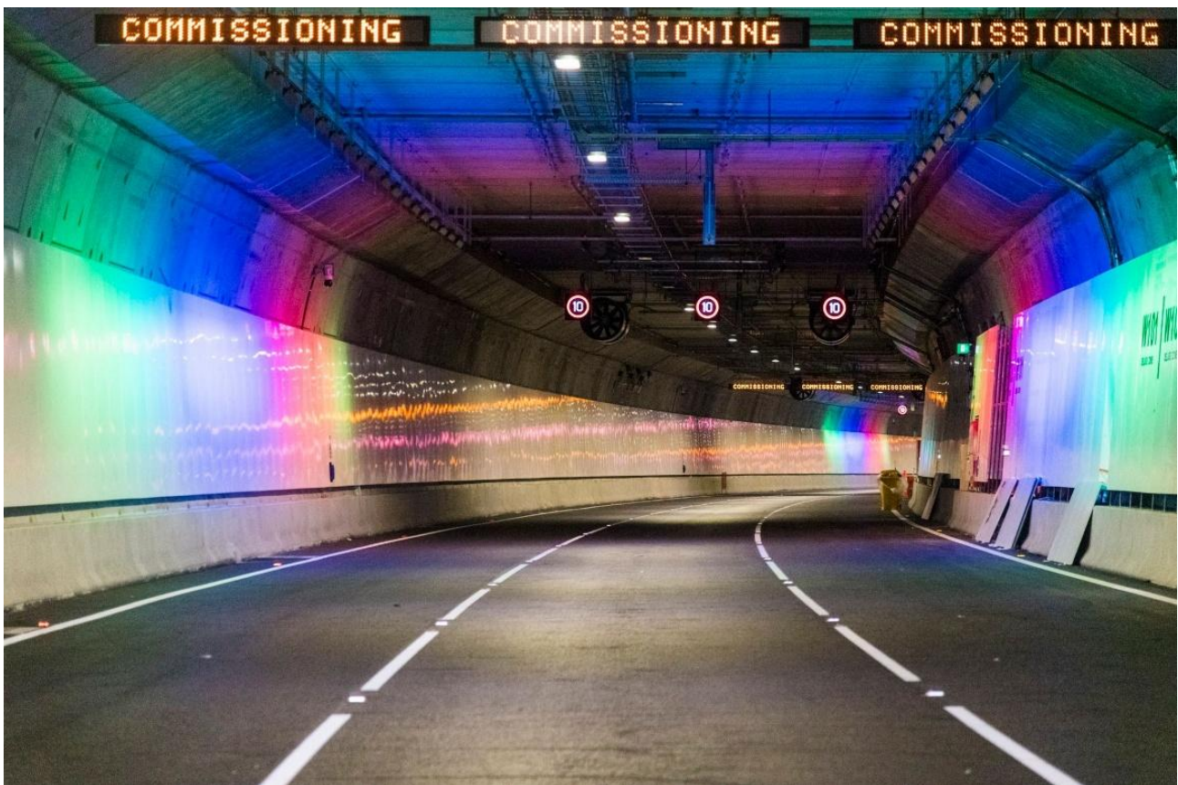
Photo 3 – Tunnel Commissioning (Source: WGTP VIDA Roads, November 2025)
