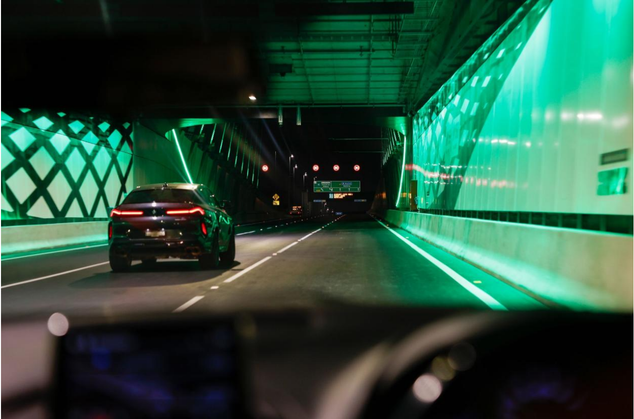
Photo 6 – West Gate Tunnel Open to Public Traffic (Source: WGTP VIDA Roads, December 2025)
