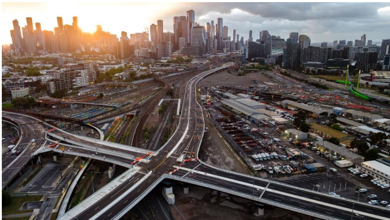
Photo 1 – Wurundjeri Way extension intersection (Source: WGTP VIDA Roads, October 2025)
