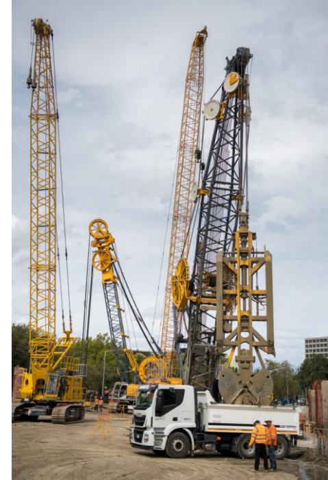
Works in the southern section of the station box
