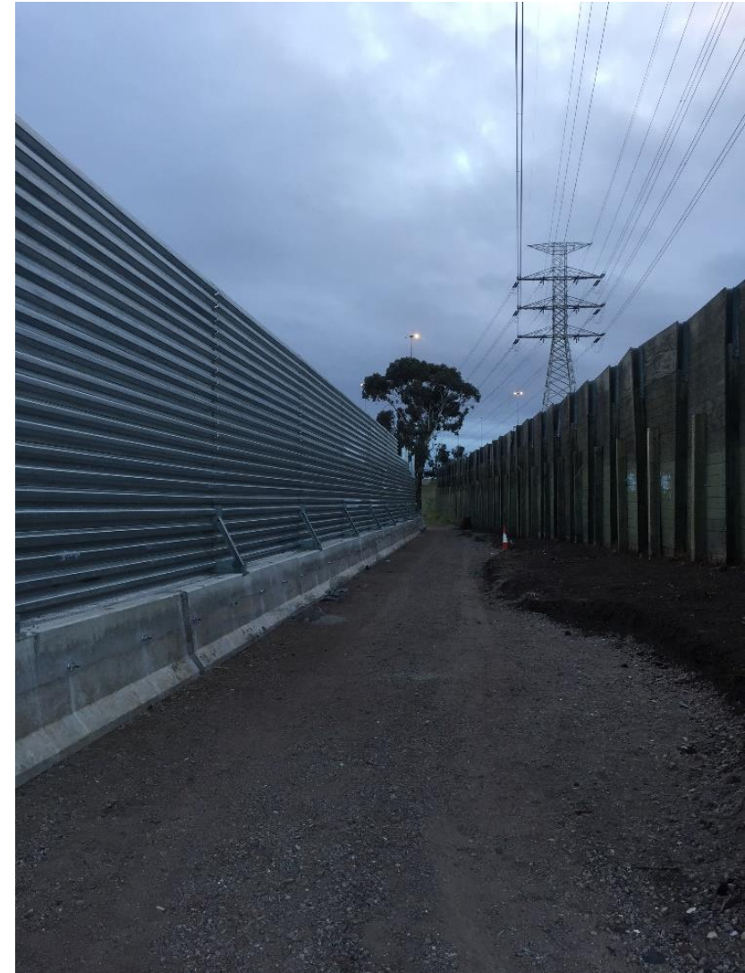
Temporary noise wall at the Williamstown Road exit ramp inbound
