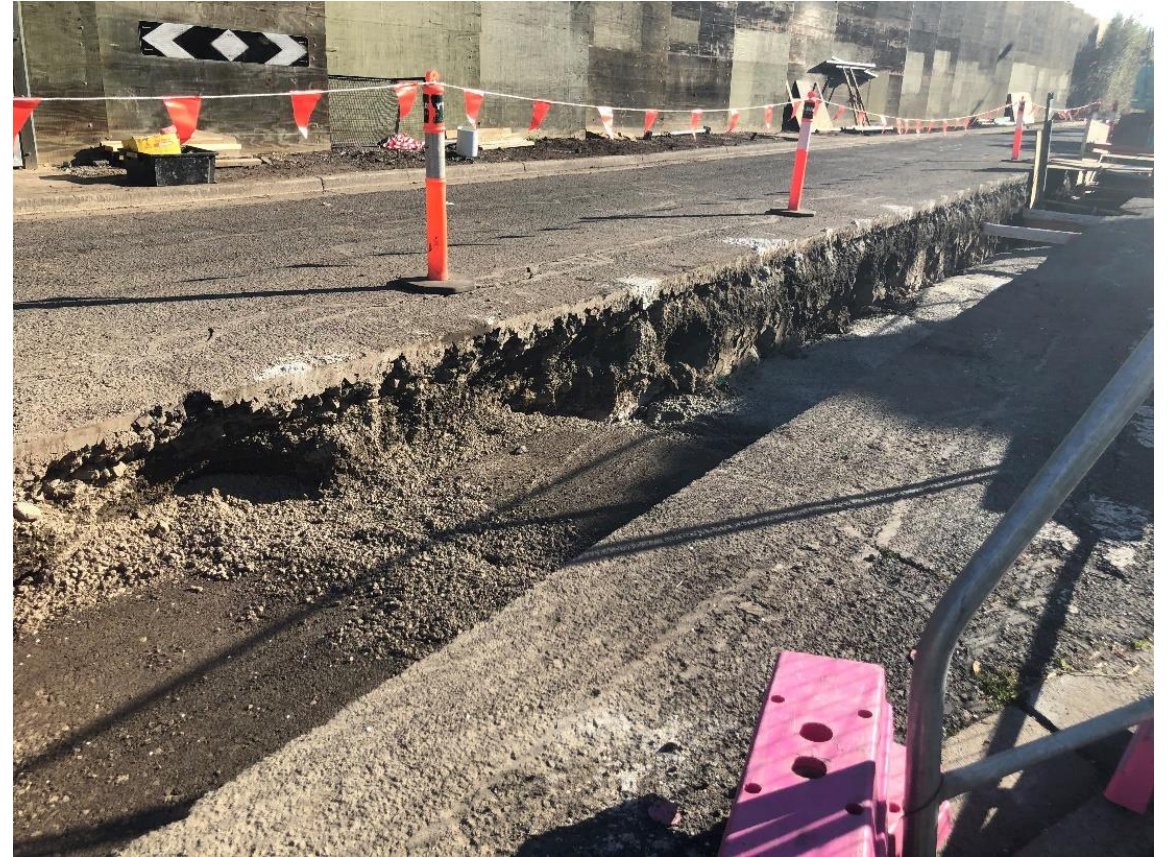
Trenching works on Fogarty Avenue
