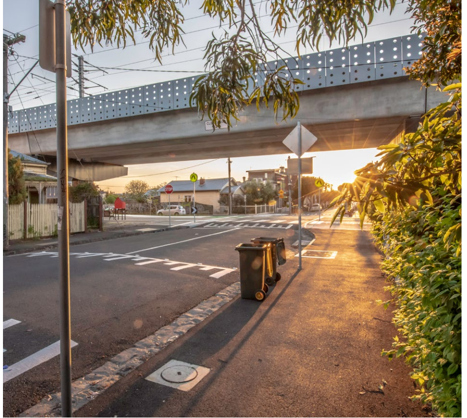
Reynard Street, part of the B2M level crossing removal project
