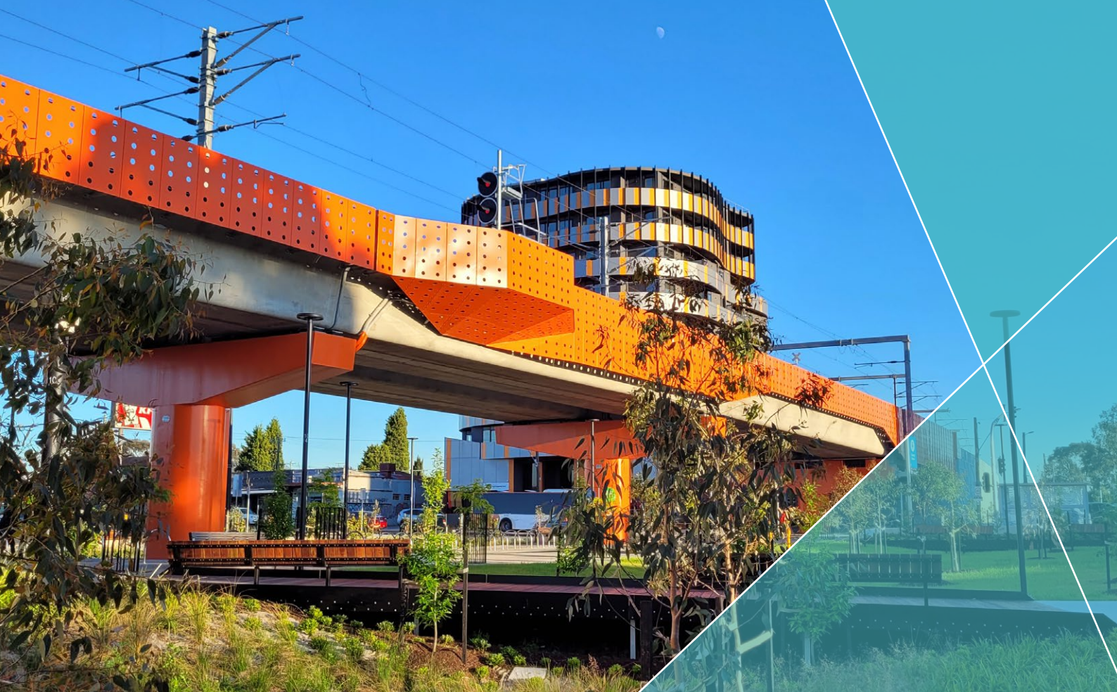
Bell Street, part of the B2M level crossing removal project
