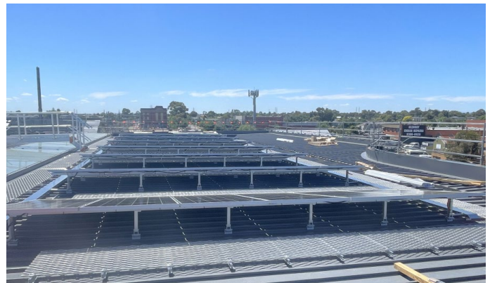
Solar Panel Installation on Concourse Roof
