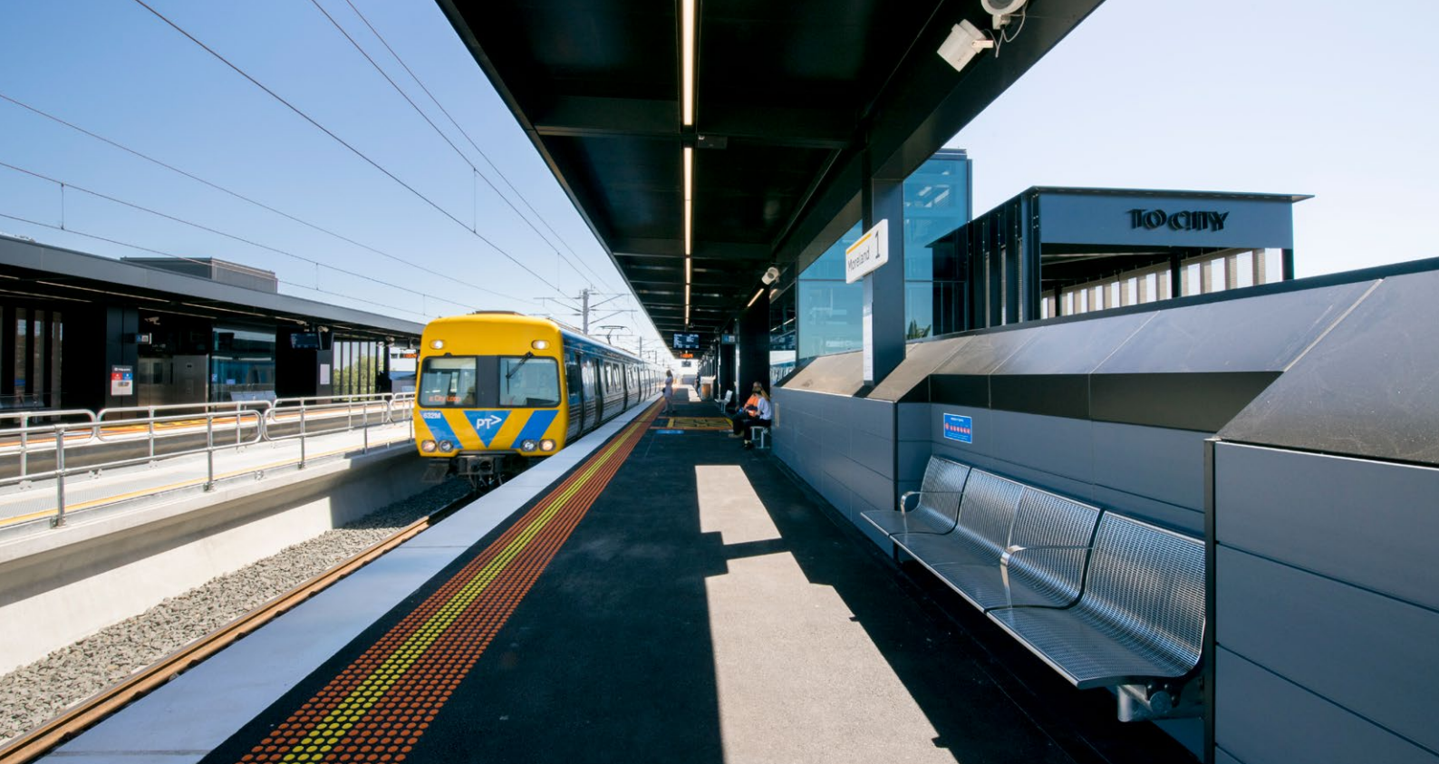
Moreland Station, Platform 1
