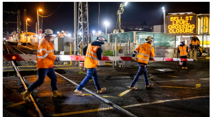
The level crossing being removed at Bell Street
