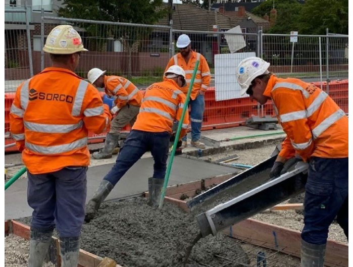
Recycled Glass Fines poured at Reservoir Station
