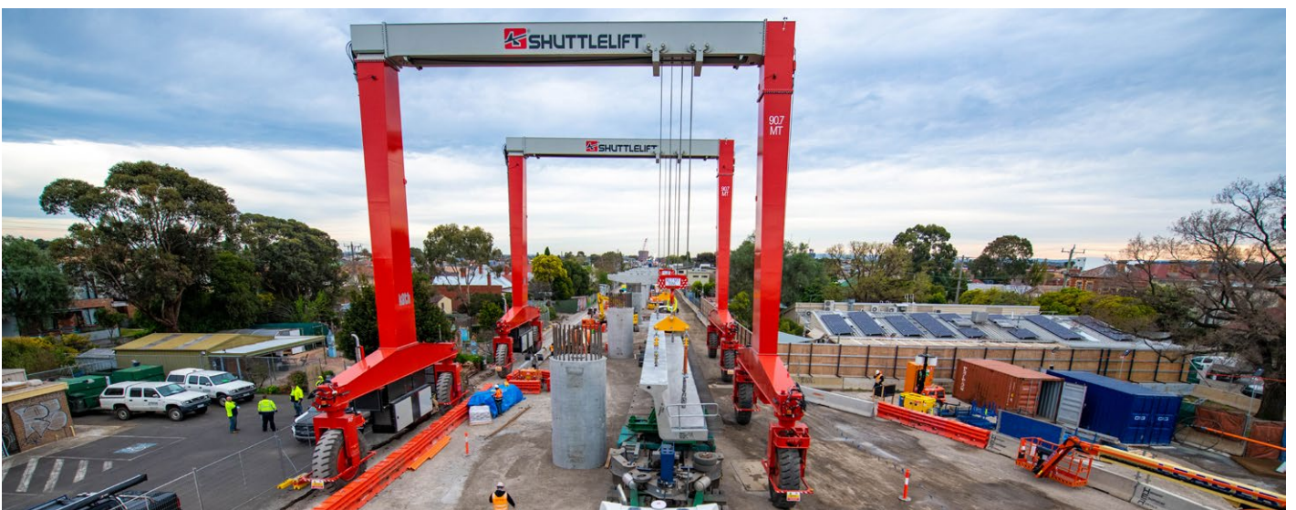
L-Beam Installation at Bell to Moreland
