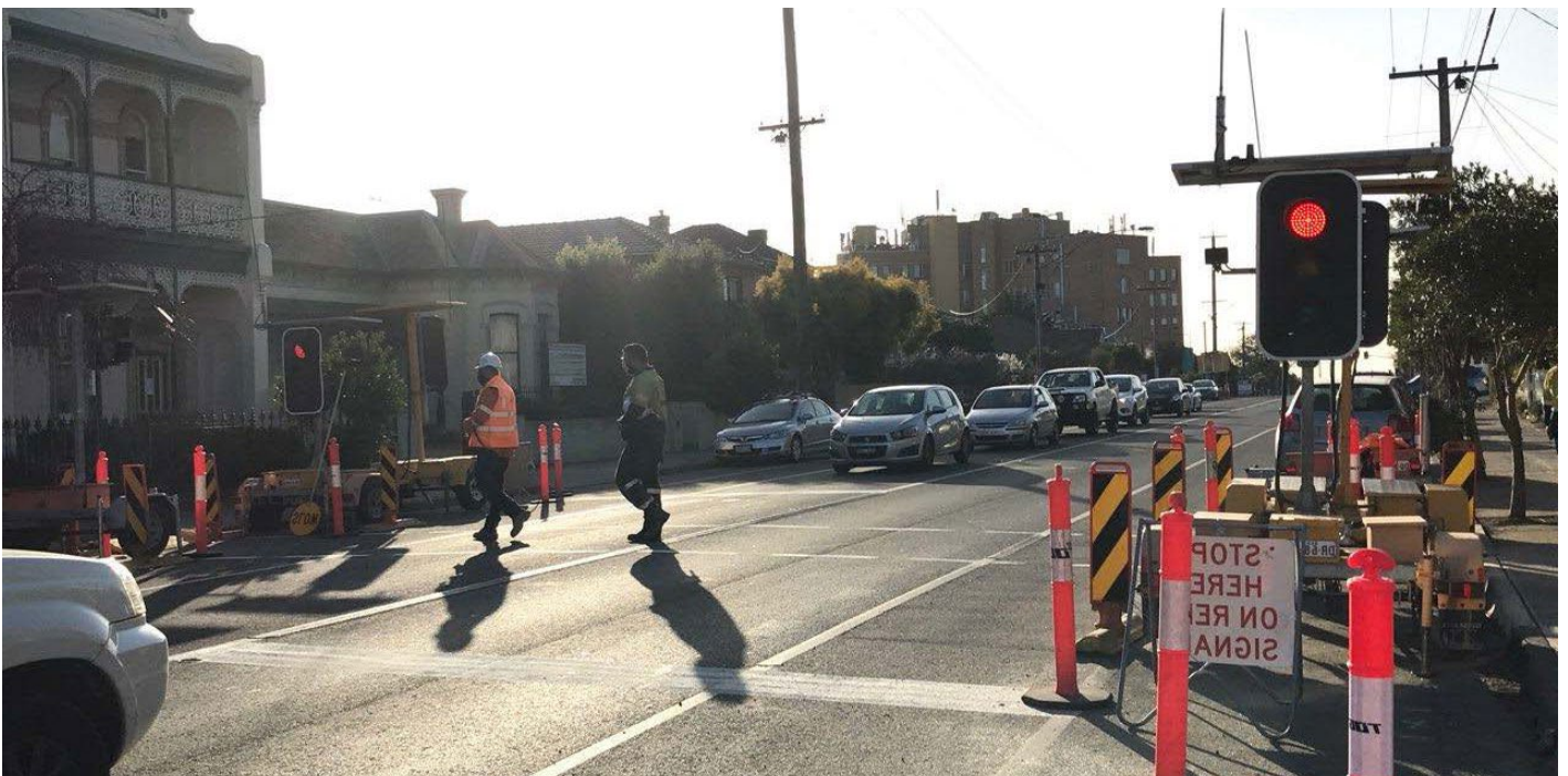
Solar Powered Traffic Lights Installed at During Bell to Moreland
