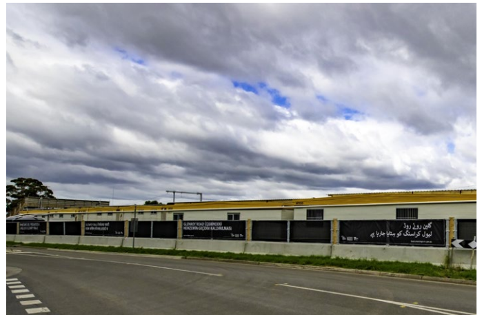
Screening and hoarding signage at Glenroy
