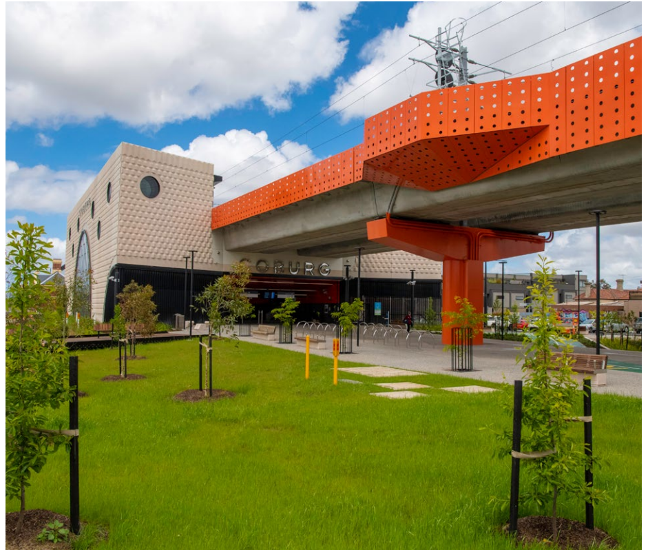
Greenery planted by YMCA Rebuild
