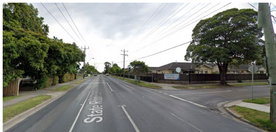
Figure A1.12: Signalised pedestrian crossing on Clayton Road
