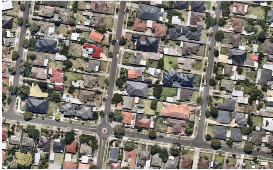
Figure A1.38: Regular residential blocks to the west of Monash University
