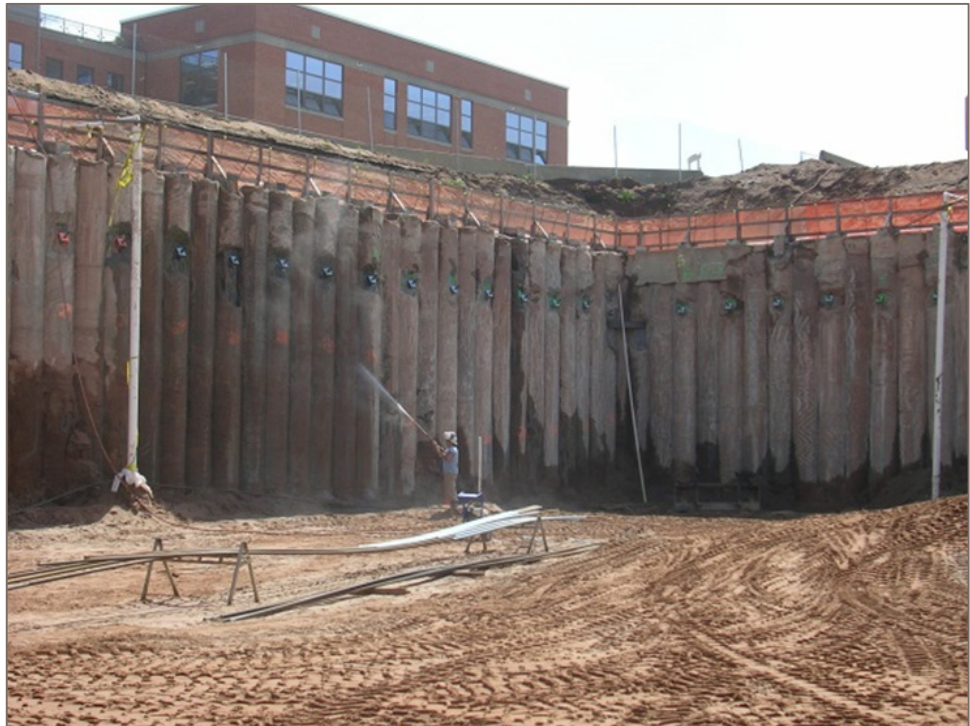
Secant pile retaining wall
