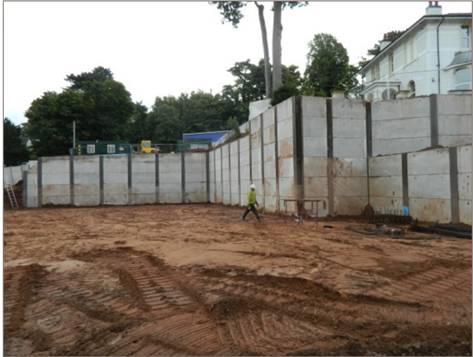
King post pile retaining wall
