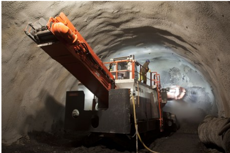
Figure 6-14 Heading excavation using a roadheader
