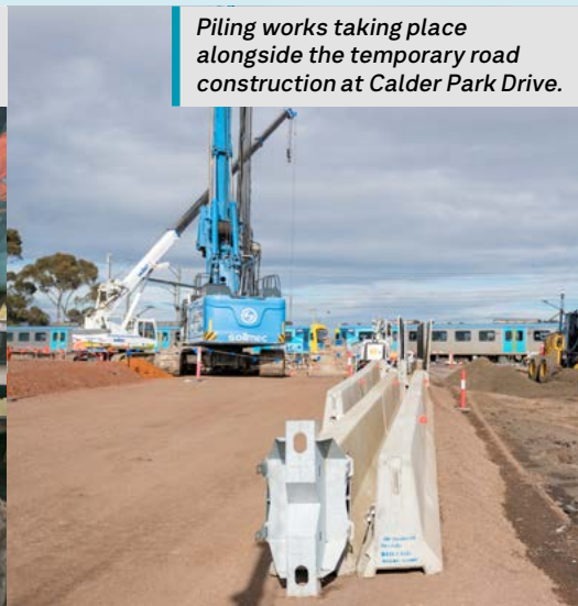
Piling works have started to build the foundations for the road bridge at Calder park Drive.
