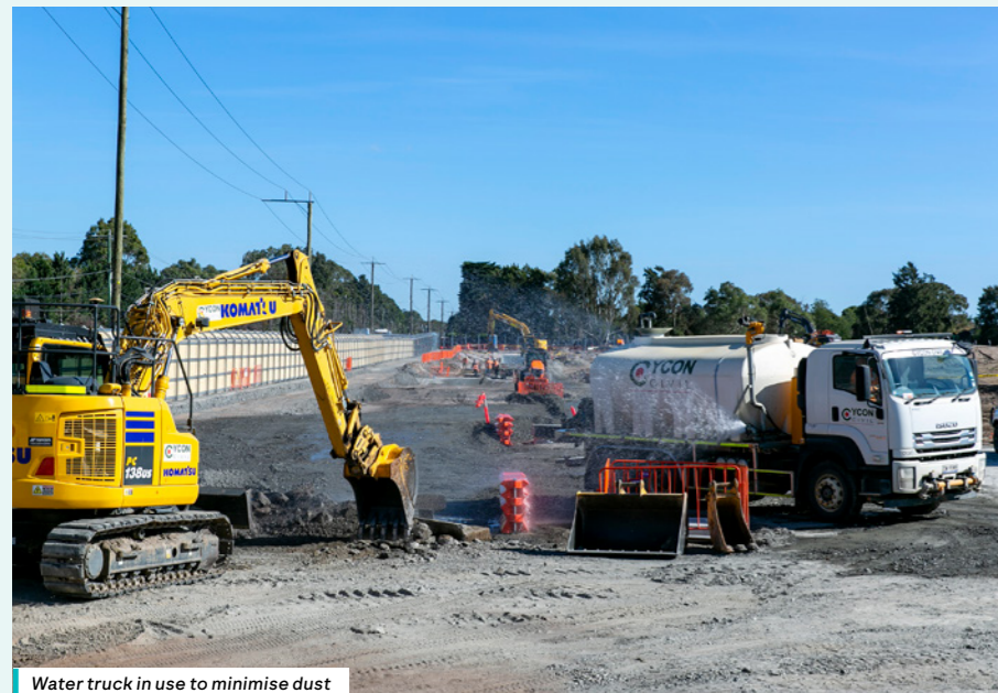
Water truck in use to minimise dust
