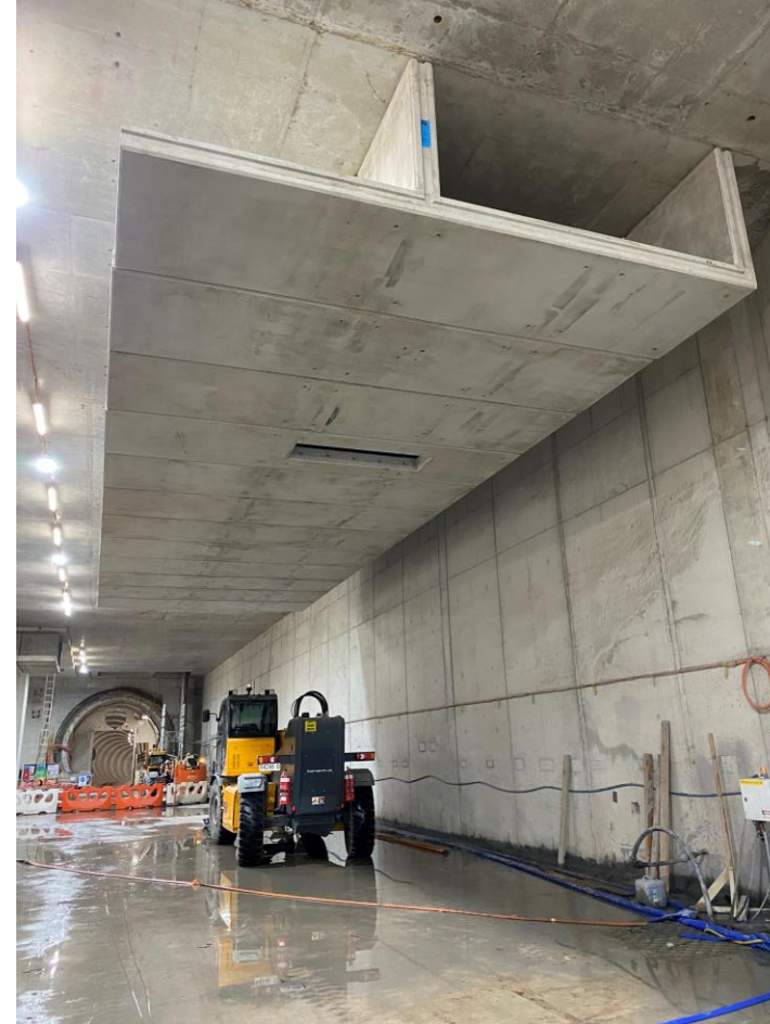
Segments of the OTE system installed in the station west box
