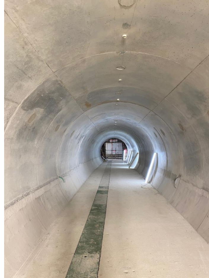
Permanent lining works complete (CP4)
