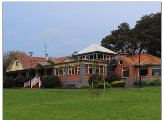
Figure 8-6 Fawkner Park Community Centre and Tennis Centre
