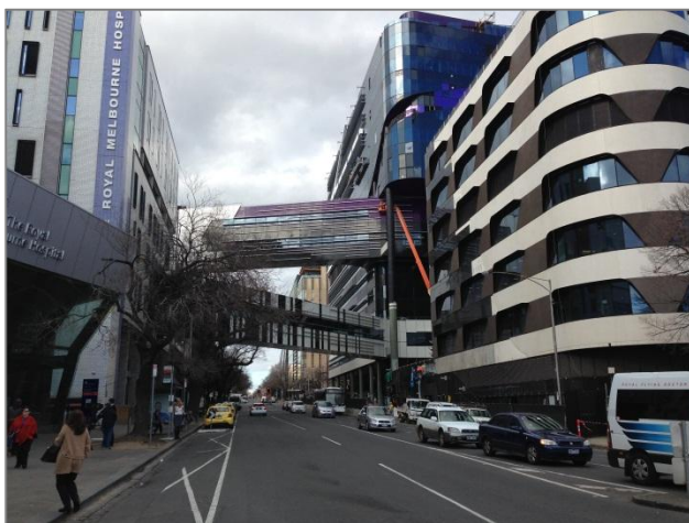
Figure 11-1 Royal Melbourne Hospital (left) and the Victorian Comprehensive Cancer Centre (right)
