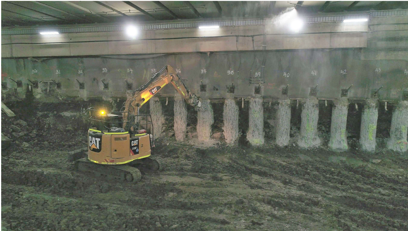
Excavation of dive structure
