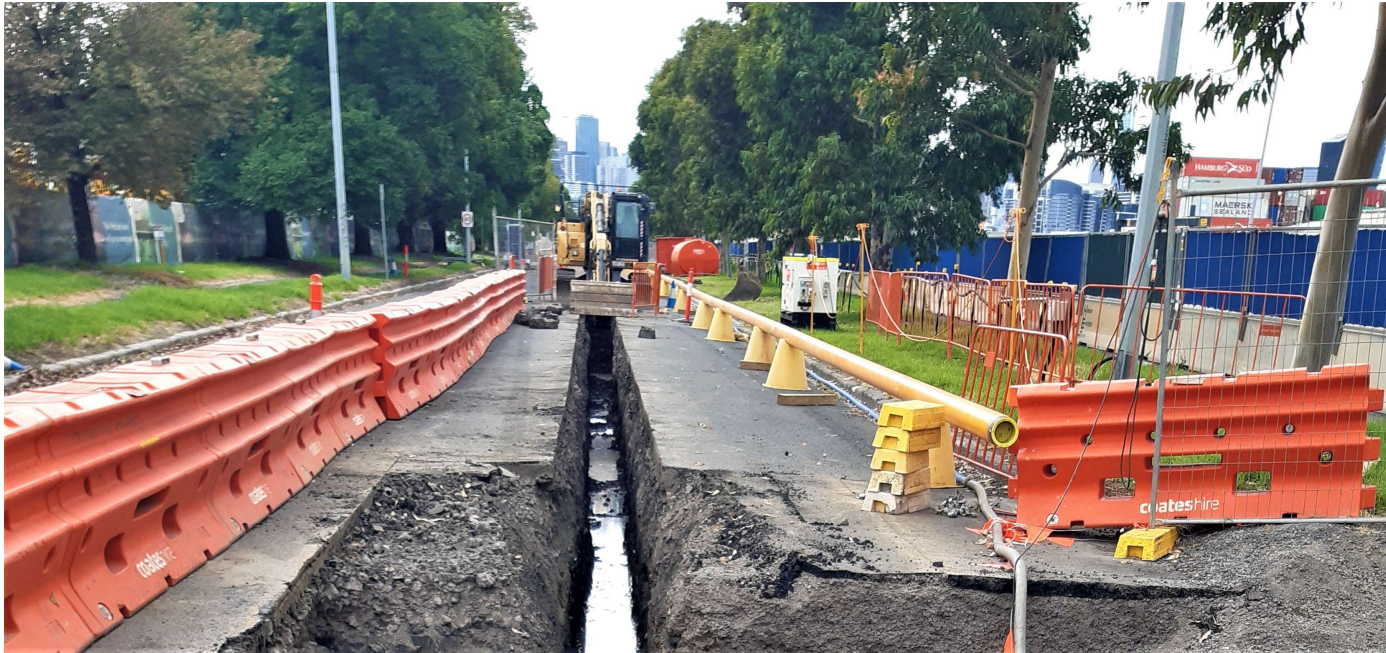
Transmission gas main relocation in the northern service lane
