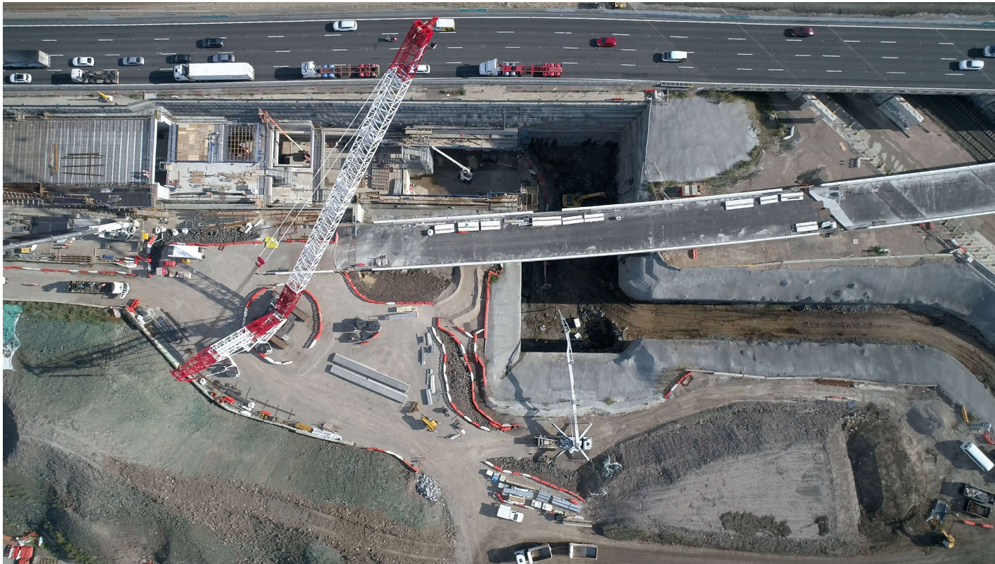
Aerial view of the Southern Outbound Portal
