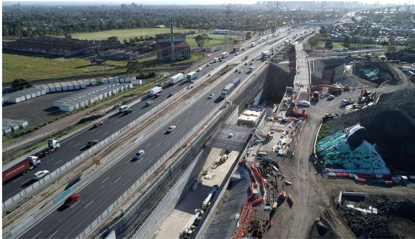
Aerial view of the Outbound Southern Portal
