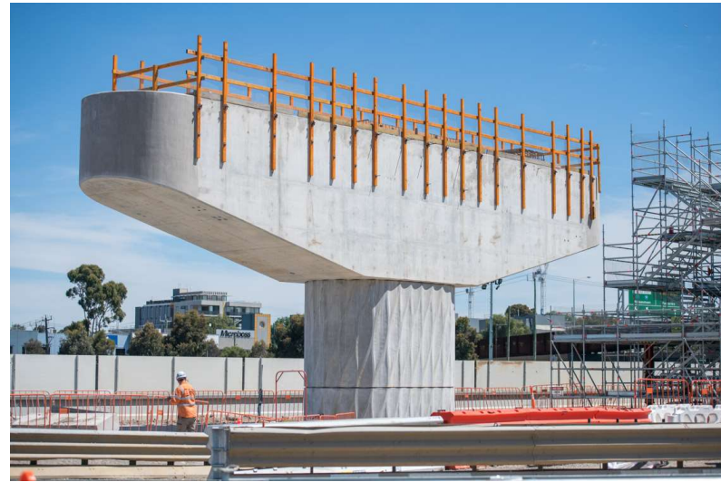
Insitu Crosshead installed
