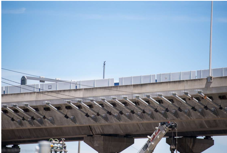
Installation of the new platforms for widening works on CityLink
