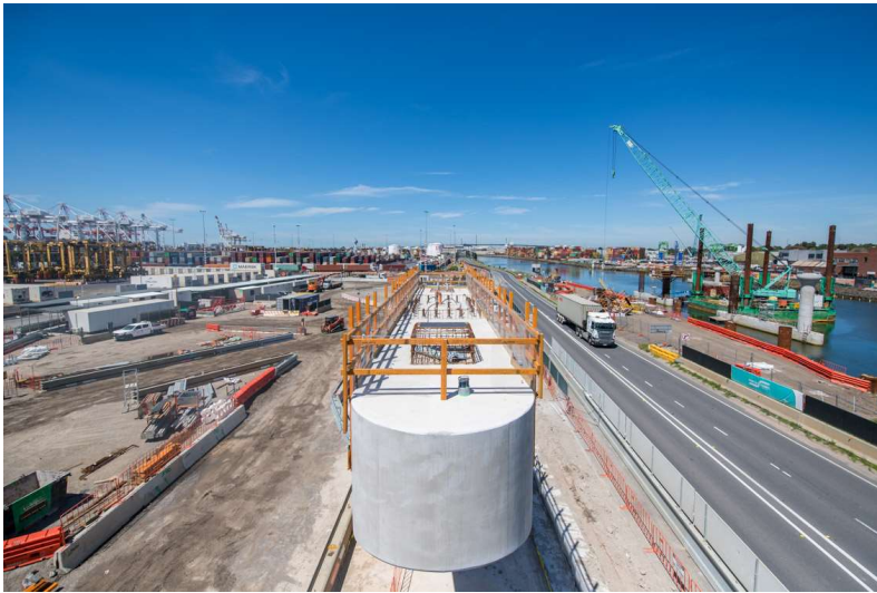
Insitu Crosshead installed
