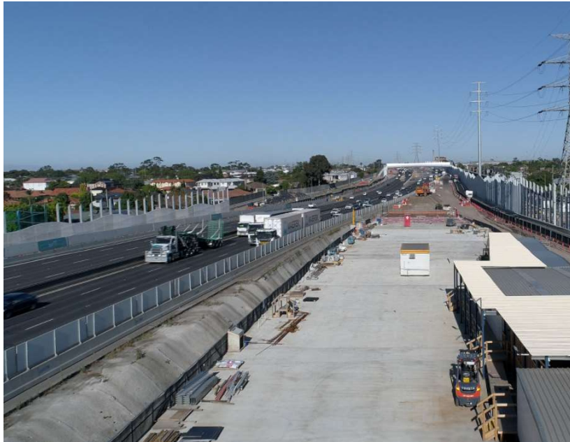
Portal roof deck looking west
