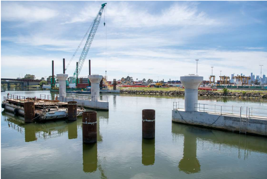
A temporary jetty for crane and bridge columns
