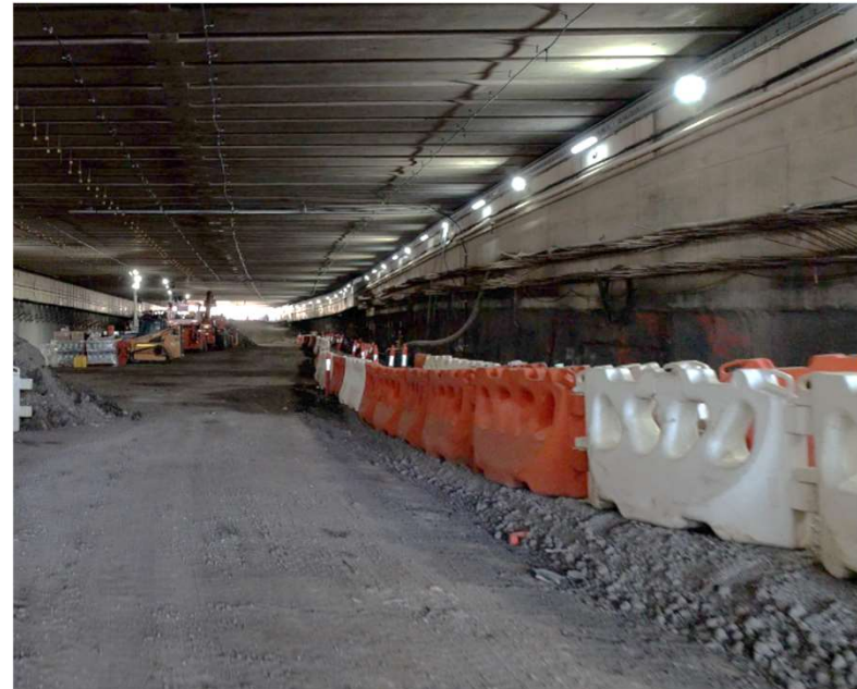
Underneath the roof deck
