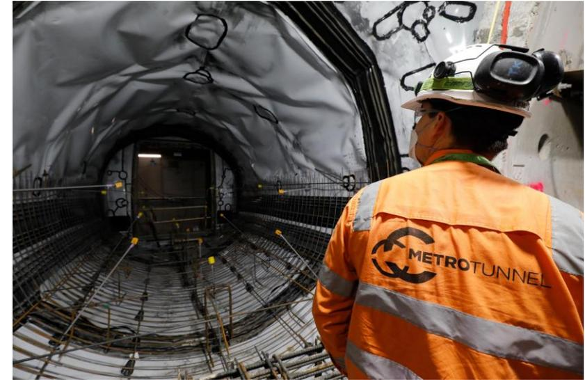
*Steelfixing installed before concrete linings can be poured*
