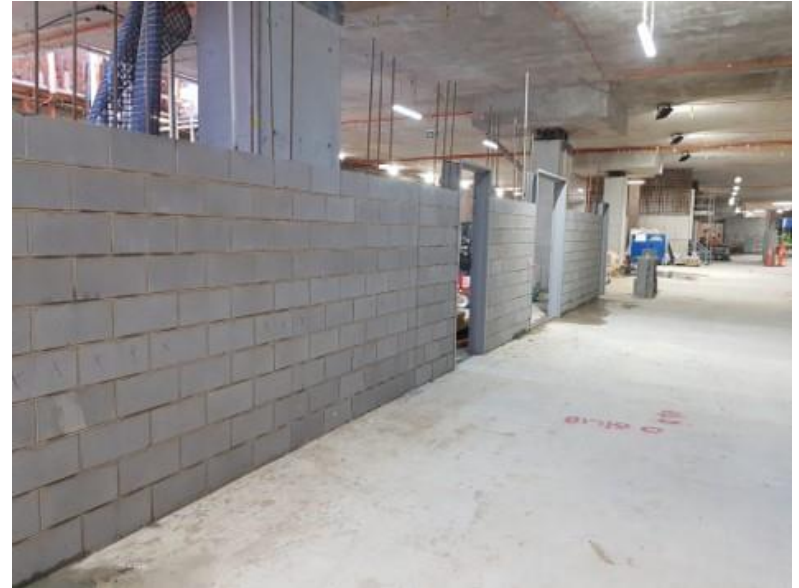
Anzac Station blockwork
