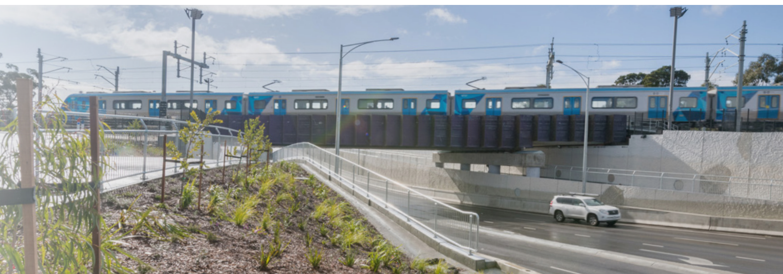
Landscaping works along Clyde Road wrapped up in July
