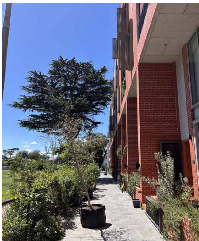
Pedestrian pathway integrated into residential development, Balfe Park, Brunswick East
