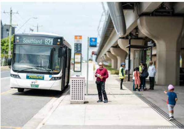
Clayton Station bus interchange
