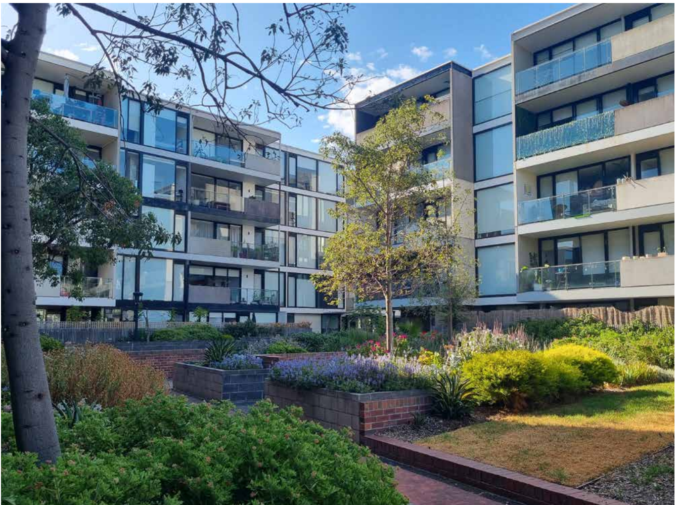
Water Sensitive Urban Design (WSUD) incorporated into mid-rise apartment development
