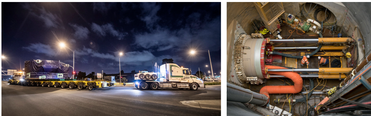
L-R: Parts of the TBM on route from the Port to the northern portal and North Yarra Main Sewer works in progress.
