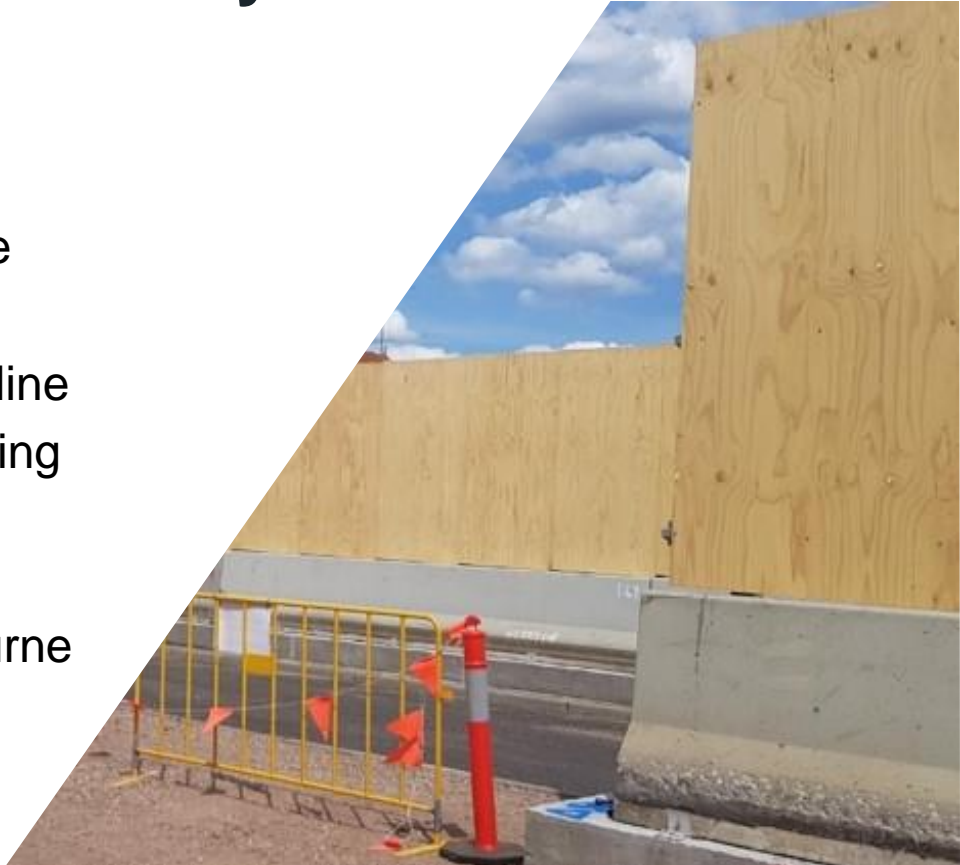
Temporary noise walls
