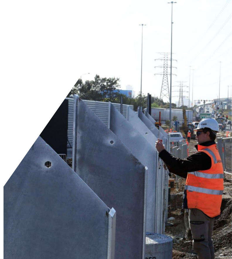
Installing foundations for the noise walls
