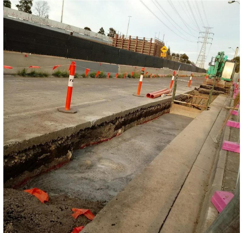
Trenching works on Fogarty Avenue
