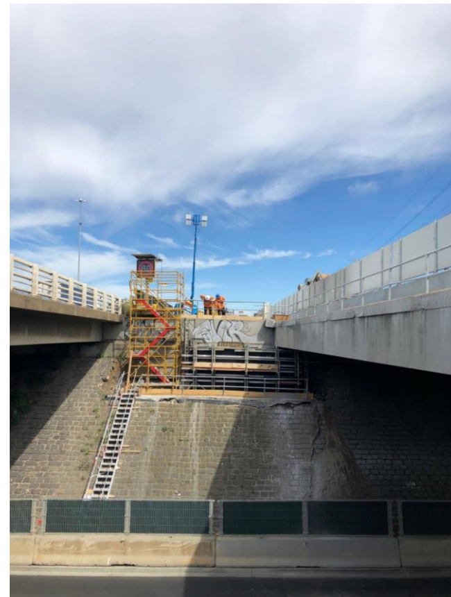
Williamstown Road freeway bridge widening works (looking West)
