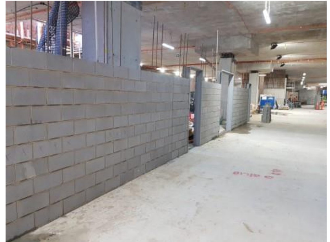
Anzac Station blockwork
