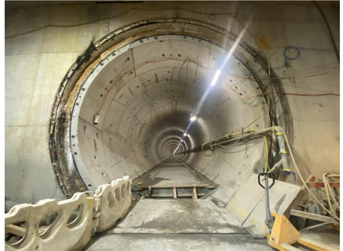
Tunnel invert completed
