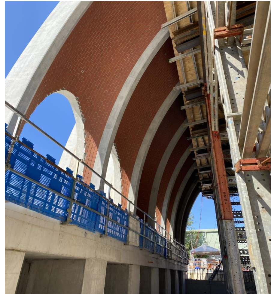
Station entrance arches being installed
