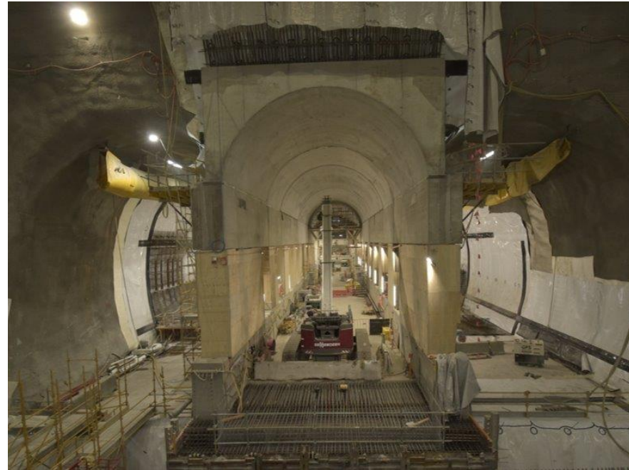
Trinocular cavern from the La Trobe Street adit
