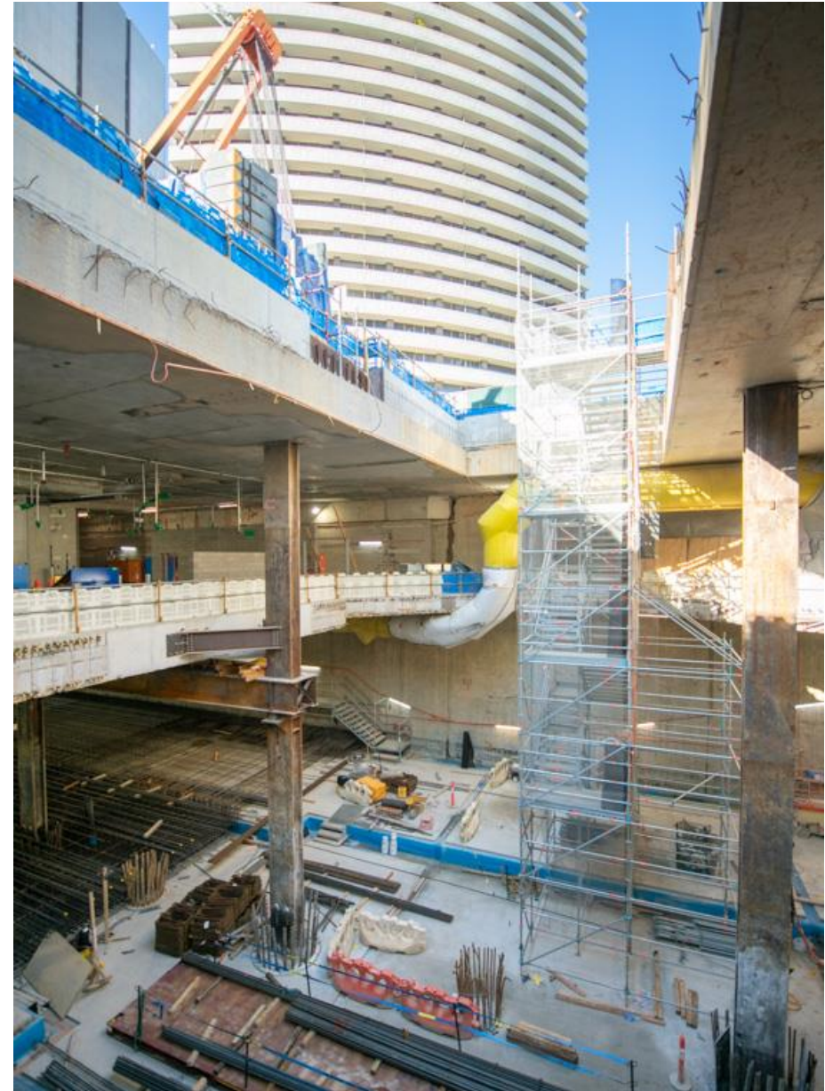
Base slab construction, concourse level and roof slab of station box
