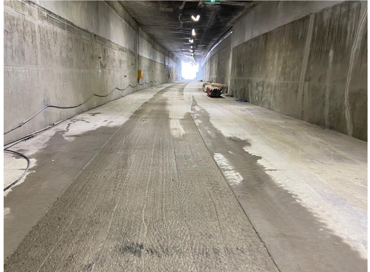
Concrete trackform in decline structure
