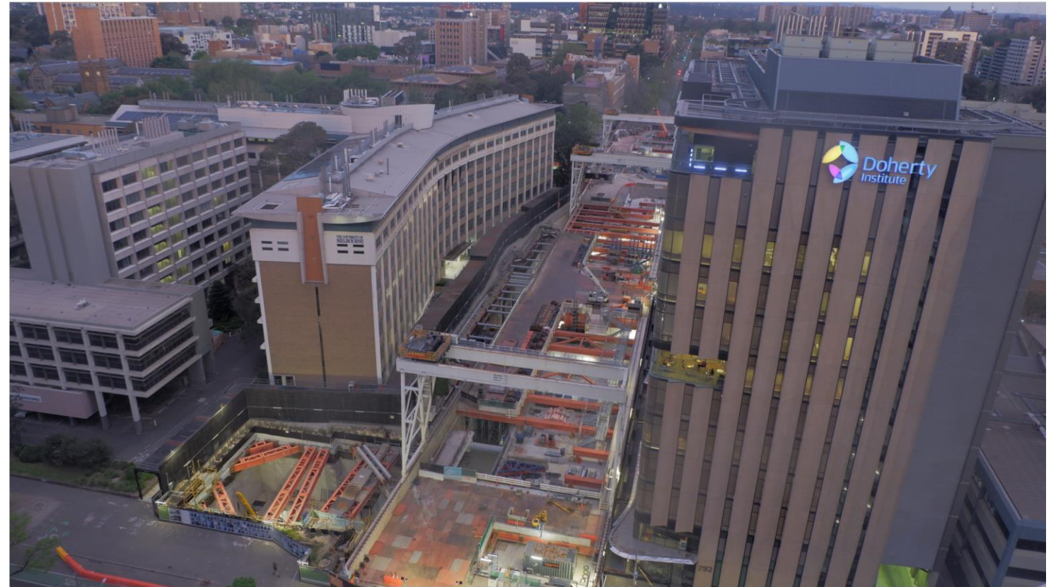
Aerial view of Grattan Street East site
