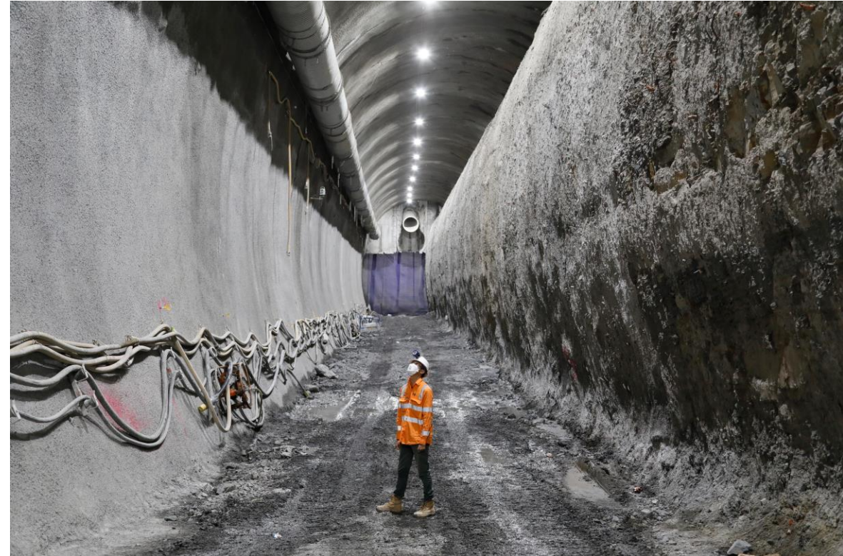
The excavated final section of the Town Hall Station Cavern
