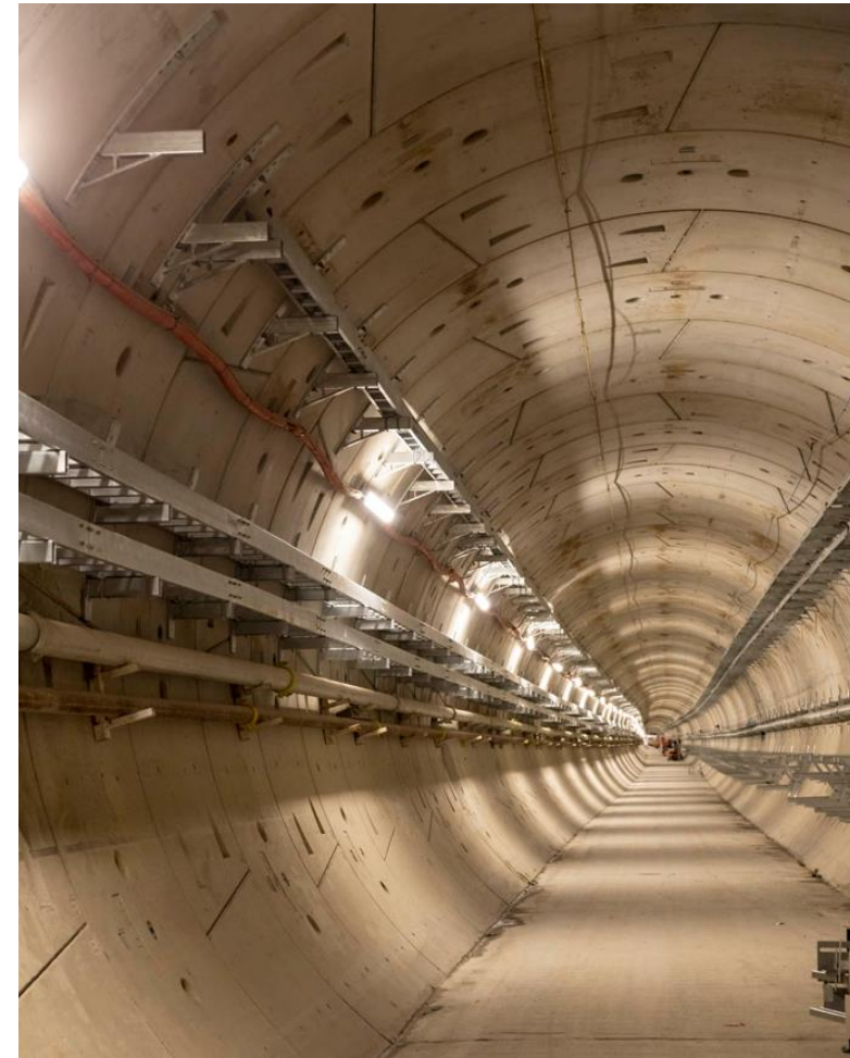
Example rail tunnel fitout works – Arden Station to Western Portal
