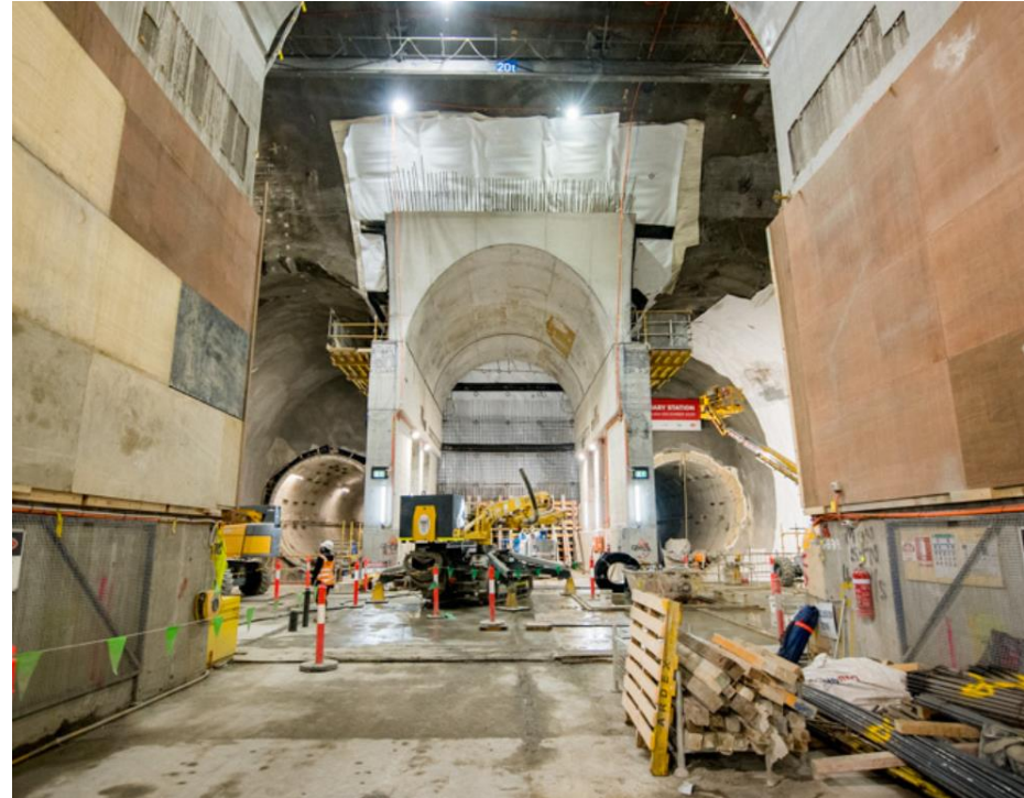
Trinocular cavern underneath Franklin Street
