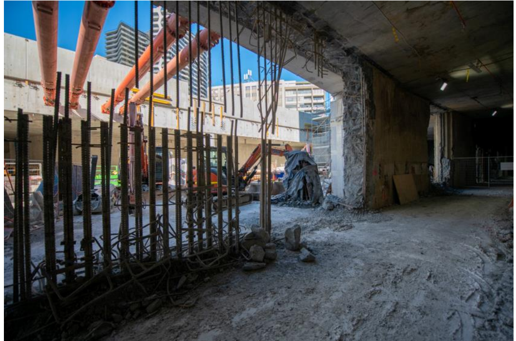
Demolished D-walls at concourse level
