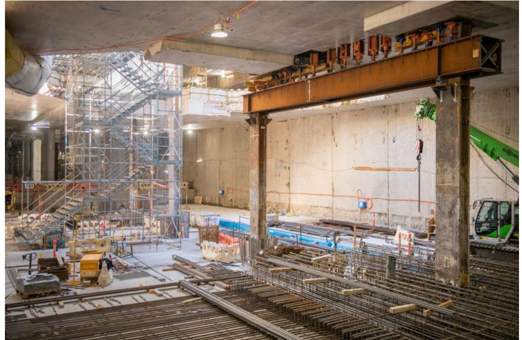
Steelfixing work for final base slab concrete pours
