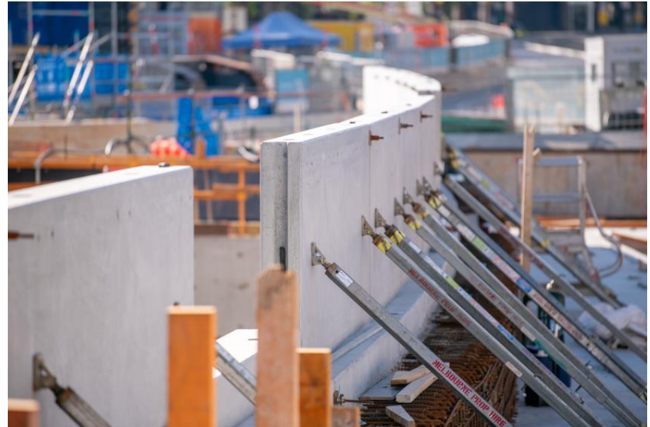
Precast panel installation at tram interchange
