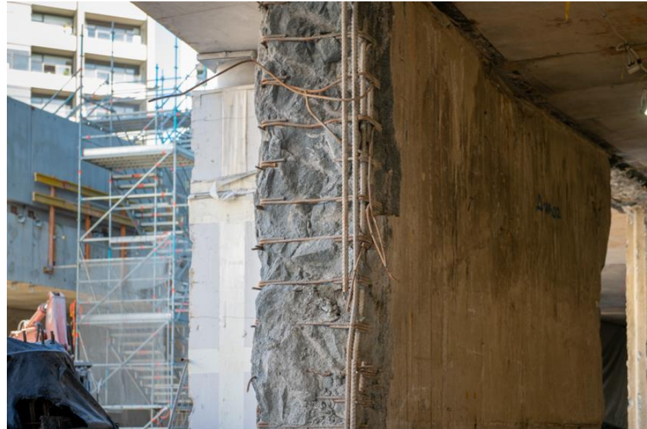
D-wall demolition – tram interchange to concourse
