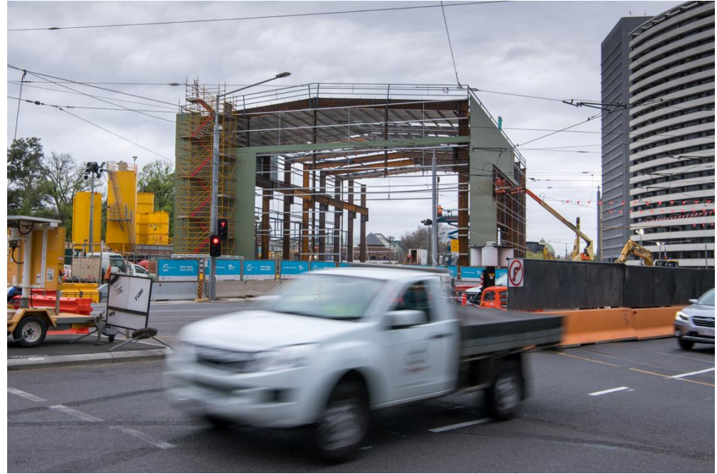
Acoustic Shed construction – October 2019
