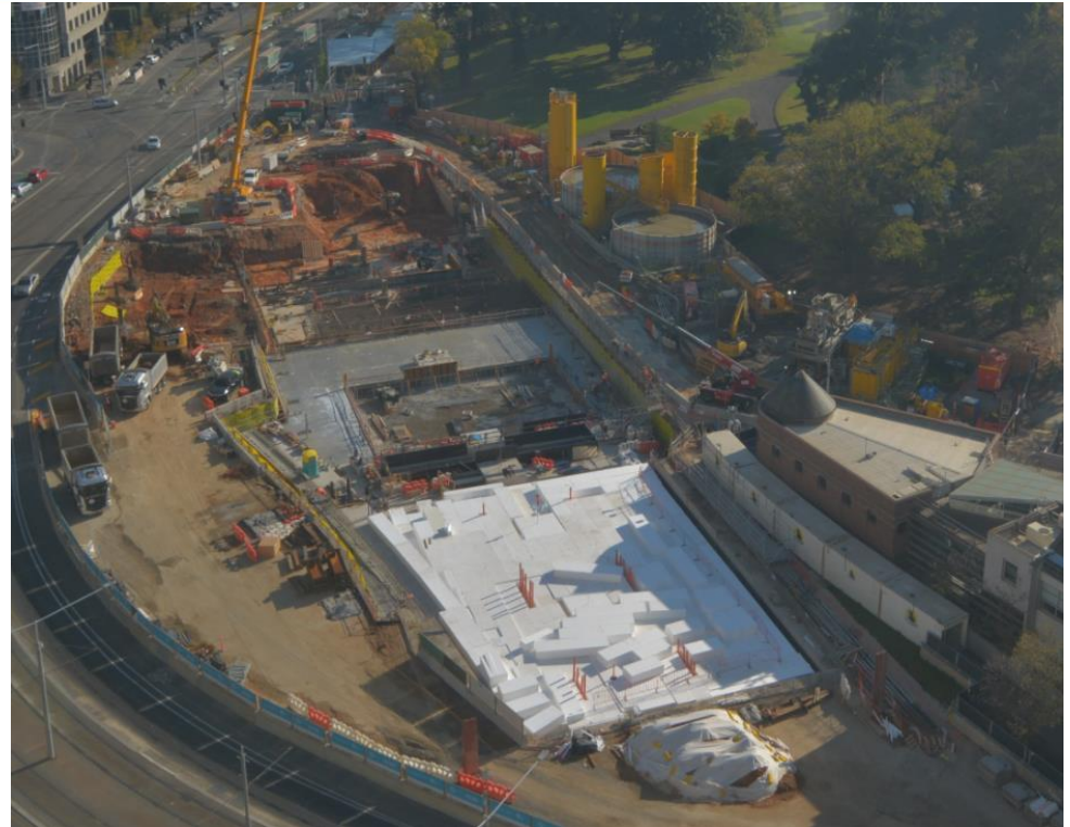
Temporary Styrofoam infill on the station roof (18 May 2019)
