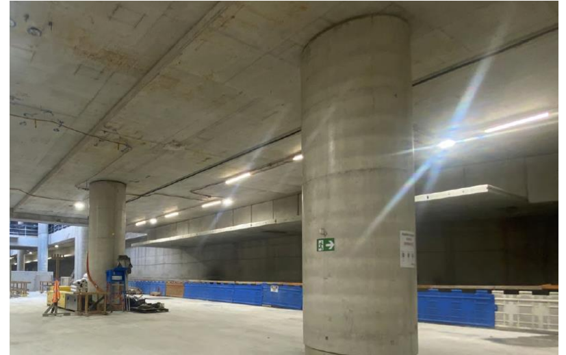
Over track exhaust installation at Arden Station
