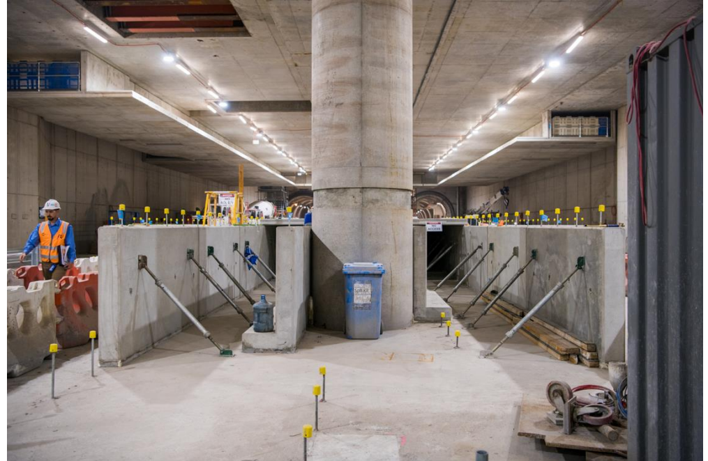
Precast panels installed at Arden, prepared for topping slab
