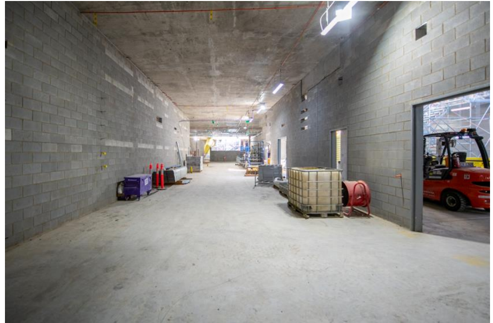
Internal rooms and blockwork at concourse level
