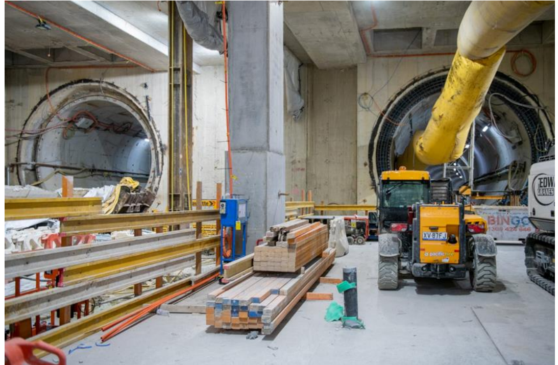
Headwall construction in northern end of station box
