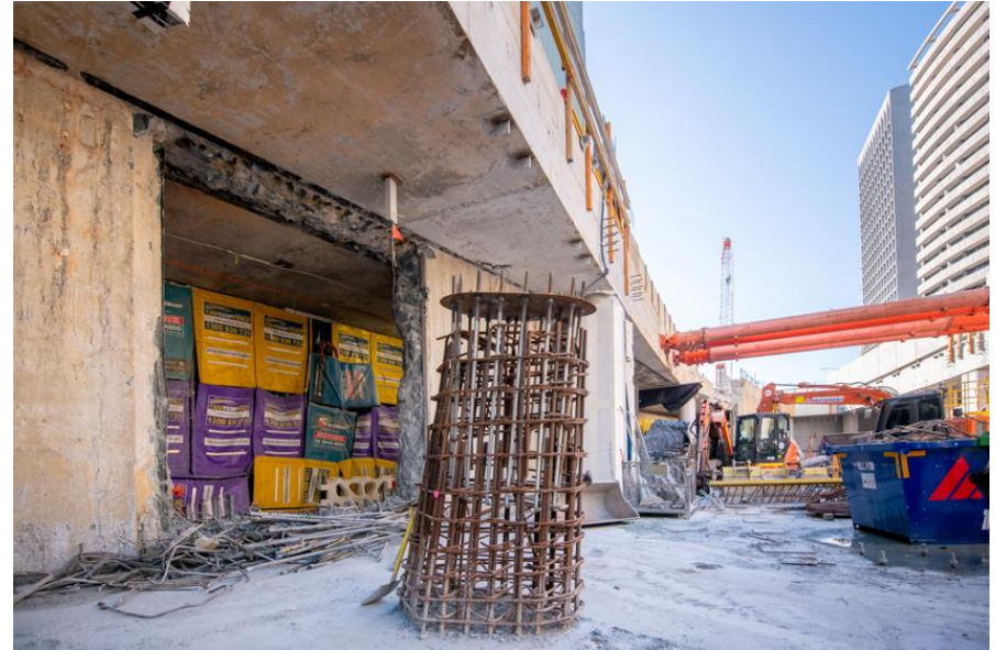
Permanent infrastructure taking shape in the tram interchange
