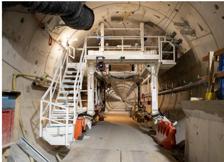
Rail tunnel fit-out gantry in use at Arden Precinct
