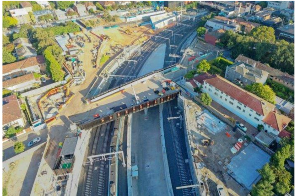
Eastern Portal decline structure
