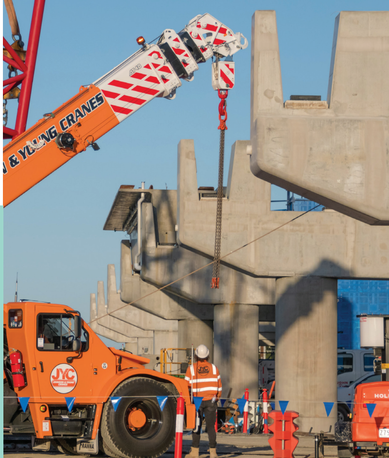
Lifting beams for the rail bridge in Pakenham
