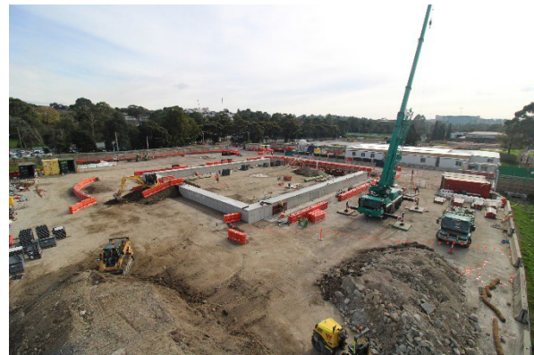
Site works at Burwood.
