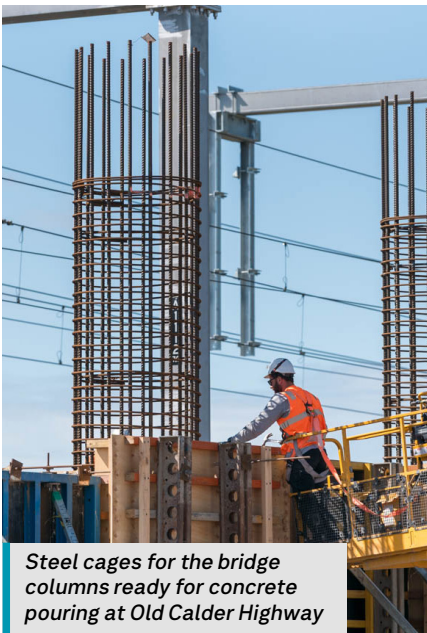
Works continuing on the pier structures for the new road bridge
