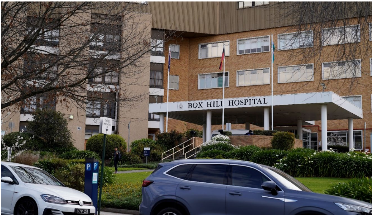
Box Hill Hospital, Box Hill
