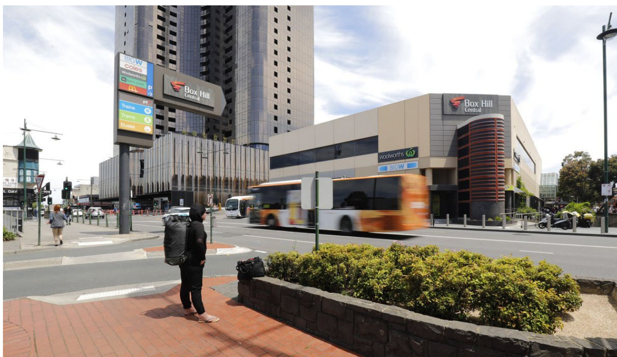
Box Hill Central Shopping Centre
