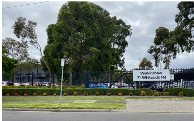
Figure A1.39: Large inward facing block
