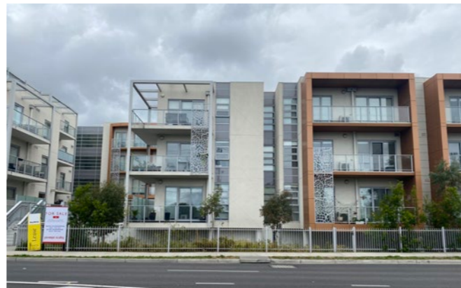
Figure A1.32: Residential building, corner of Centre Road and Clarinda Road.
