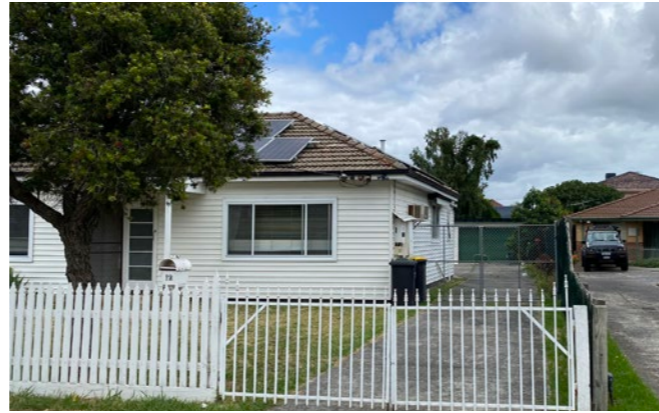
Figure A1.31: Original 1950s post-war dwelling in Clayton.
