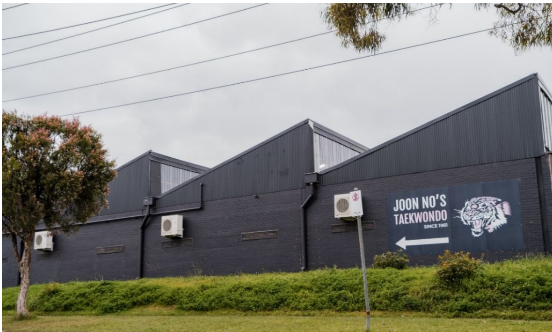
Aristoc Road building
