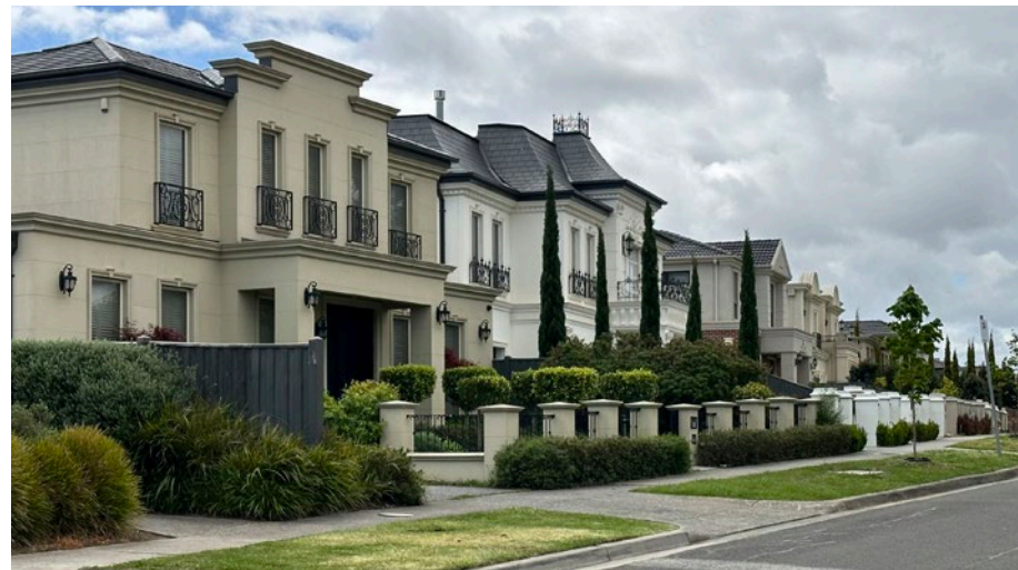
Single detached residential building
