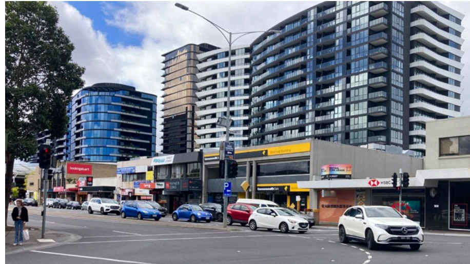
New residential apartment buildings
