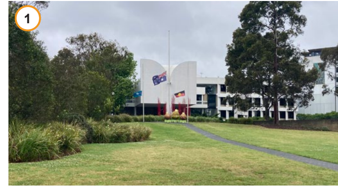
Springvale Road facing heritage item (Monash Civic Centre)
