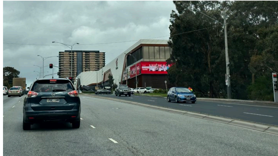
The Glen is prominently located at the high point of Springvale Road
