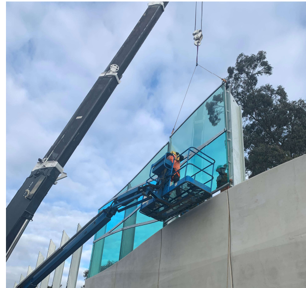
New acrylic panels expected to be installed from March
