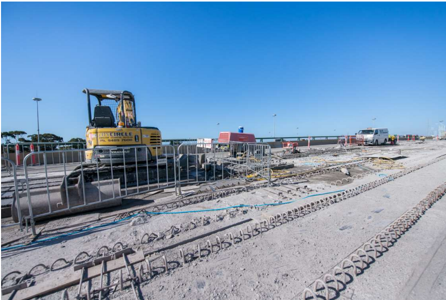
Demolition of existing road surface and pouring the concrete for new road surface
