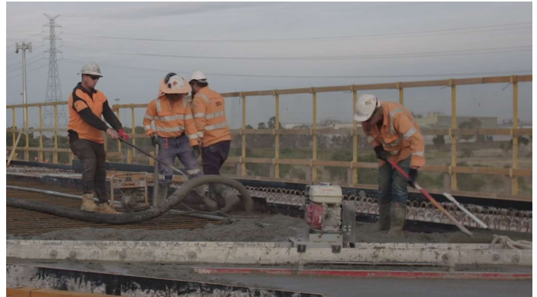
Demolition of existing road surface and pouring the concrete for new road surface
