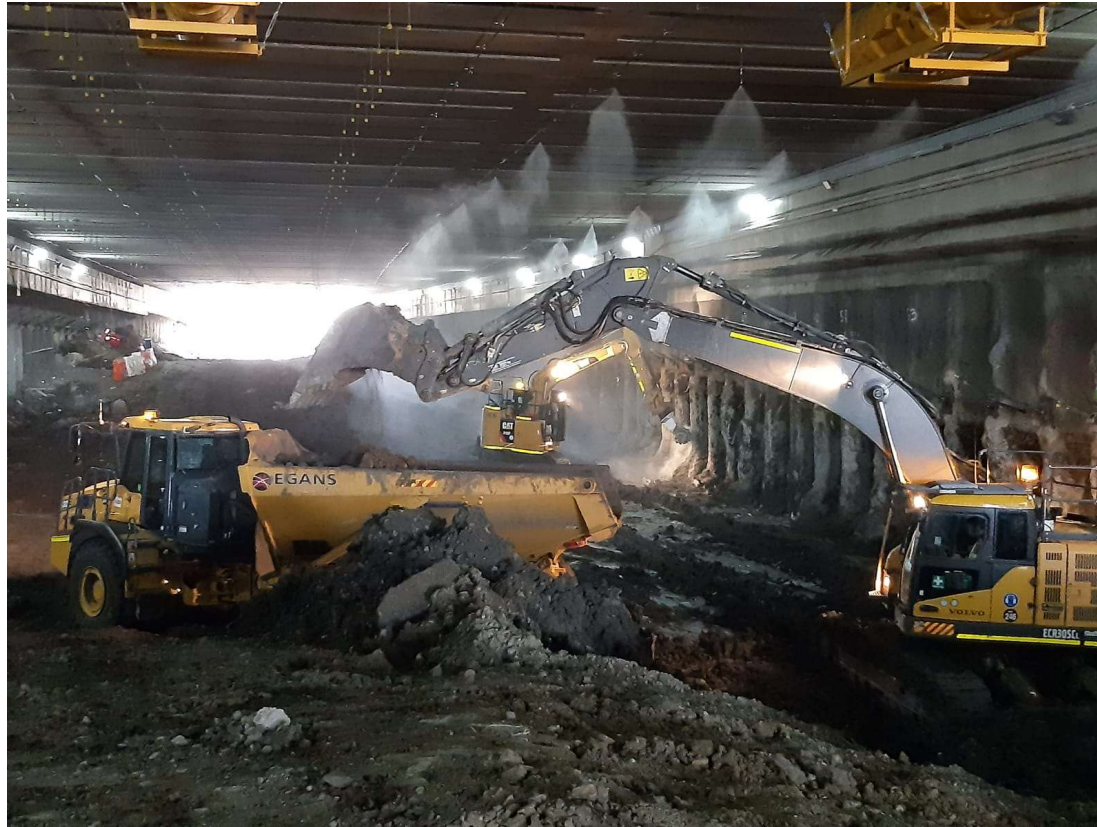
Excavation under the portal roof deck continues
