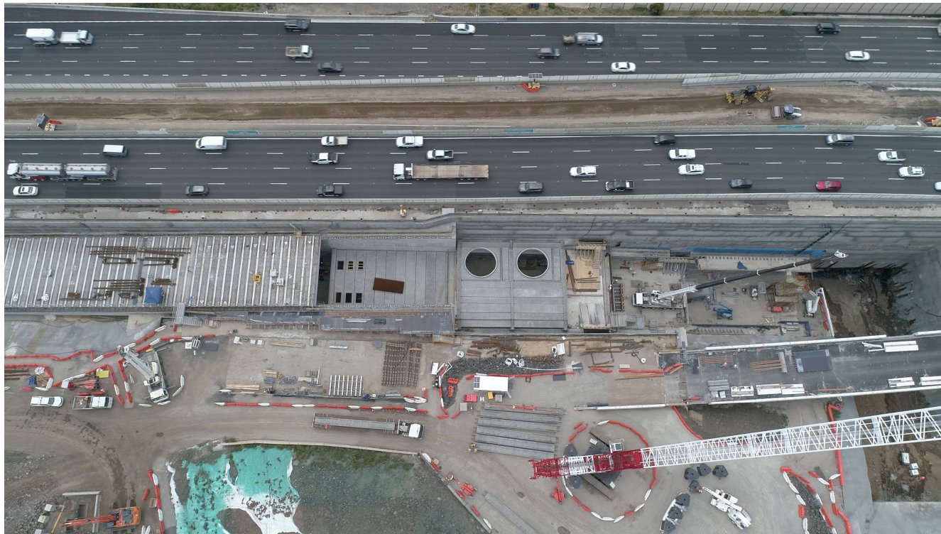
North facing aerial of southern outbound portal
