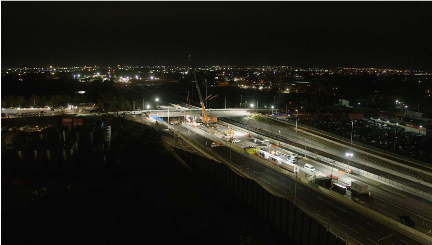
Lifting the new concrete beams into place which will become the new bridge – end of January 2021
