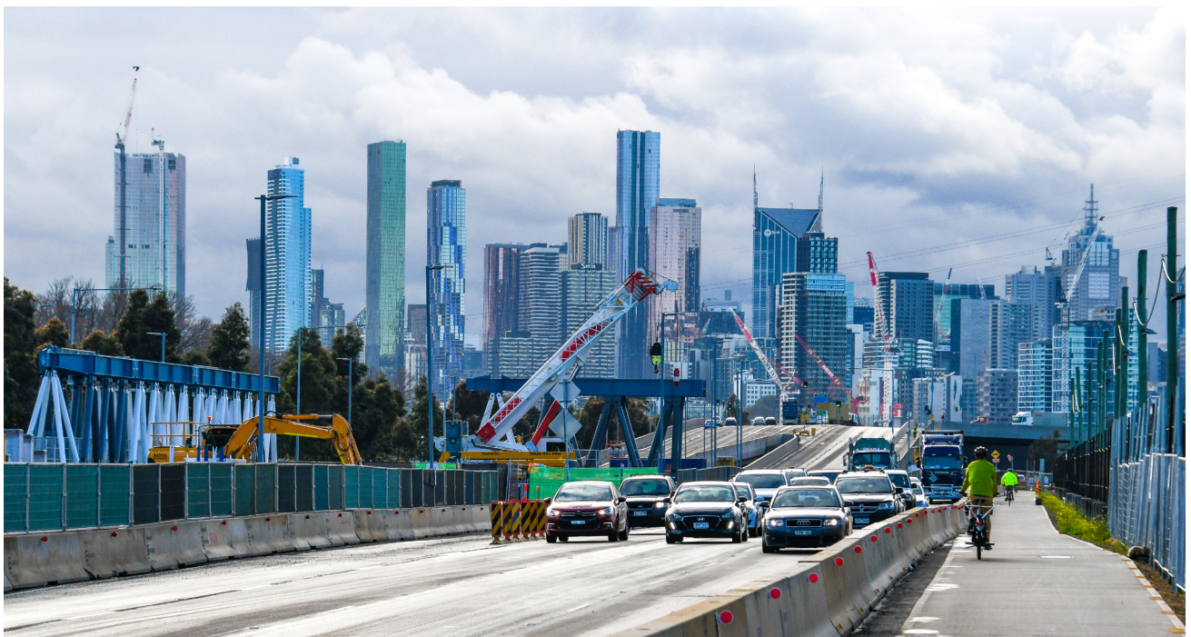
Figure 1: Launching Gantry on the Footscray Road centre median work zone
