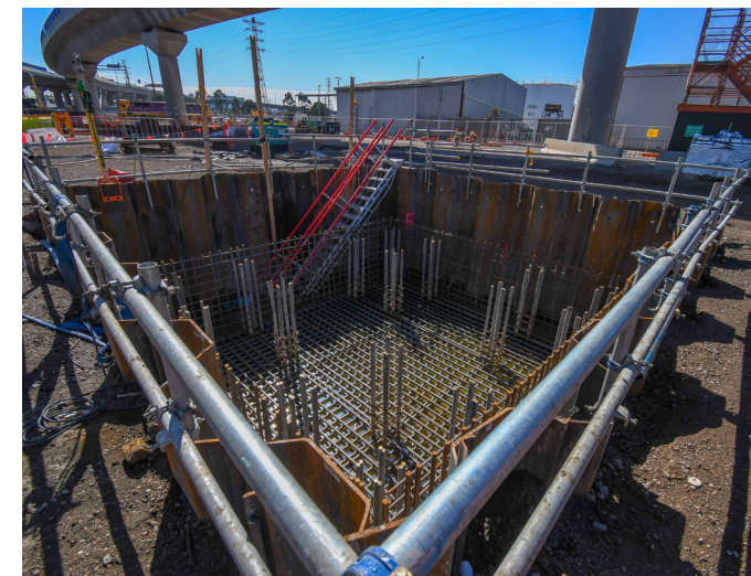
Figure 3: A pile cap ready for concrete to be poured
