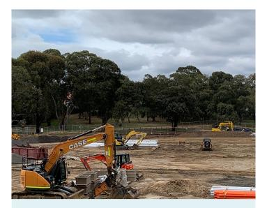
Work crews have begun excavating the existing oval at Binnak Park by removing soil and other materials, making way for the new oval and the construction of the pavilion.
