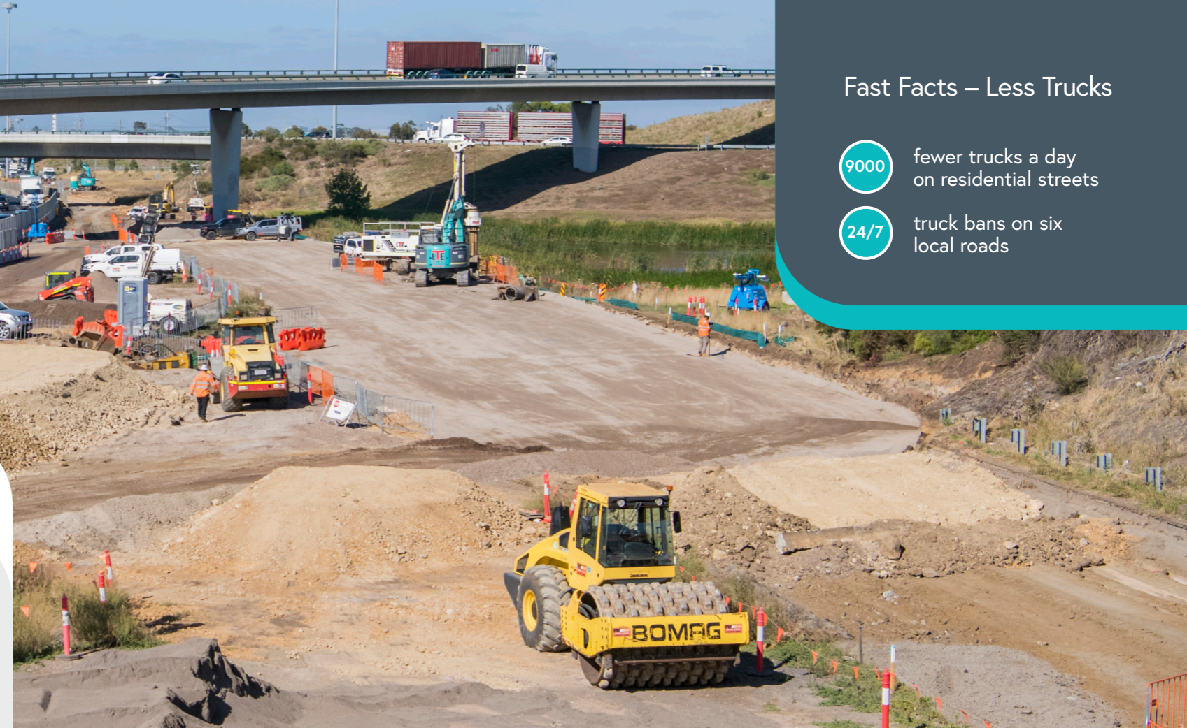
Geelong Road off ramp realignment works.
