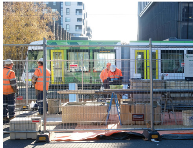
SRL East site investigations at Box Hill
