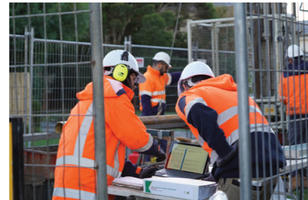
SRL East site investigations at Glen Waverley
