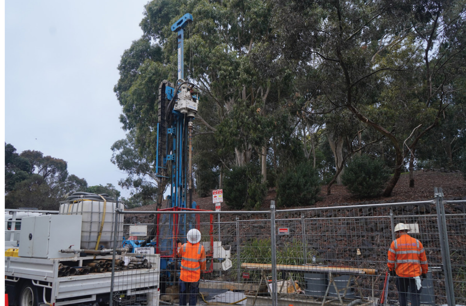
SRL East site investigations at Monash
