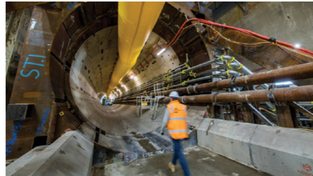
Inside Melbourne's Metro Tunnel
