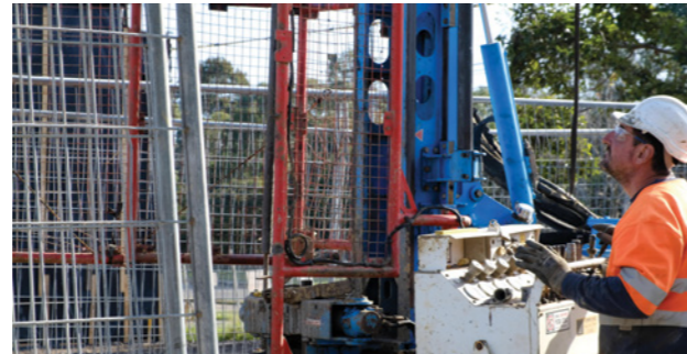
SRL East site investigations at Burwood
