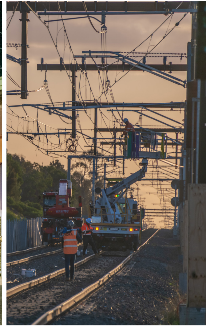
Overhead works west of McGregor Road.
