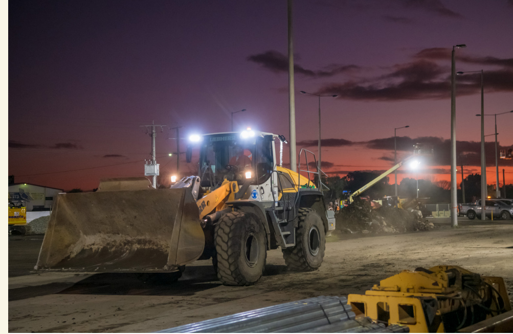
Hardstand construction works at Pakenham Station
