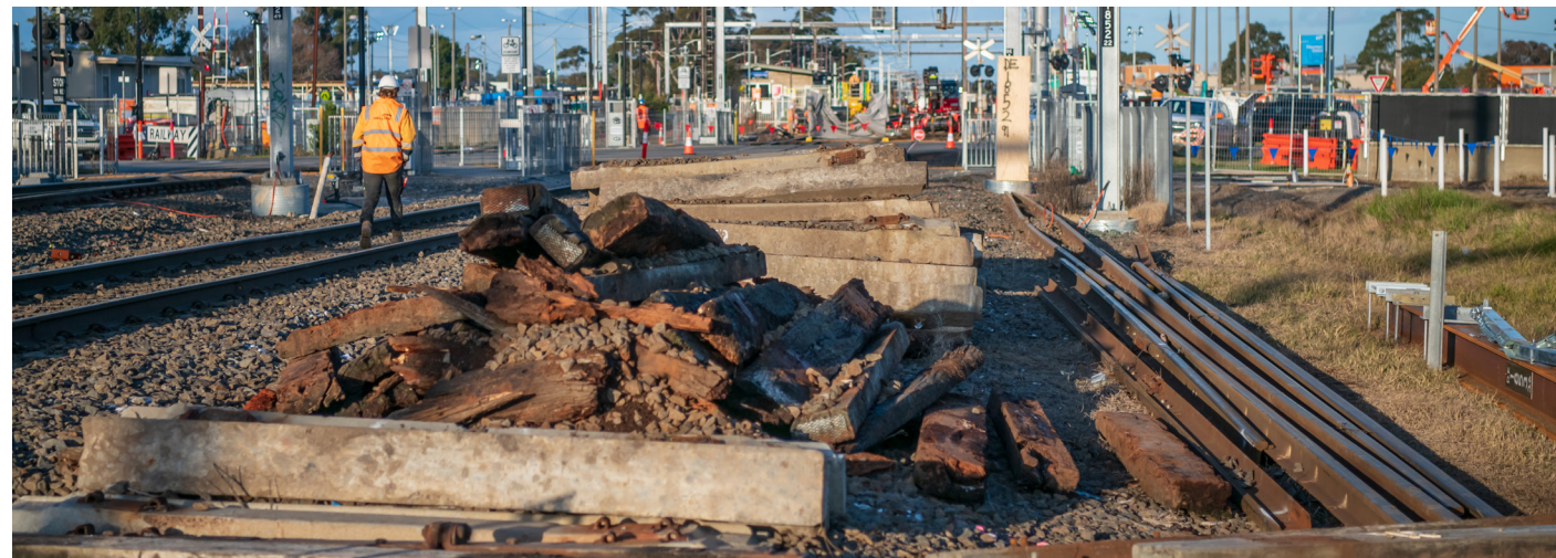
Removing track and sleepers at Main Street level crossing
