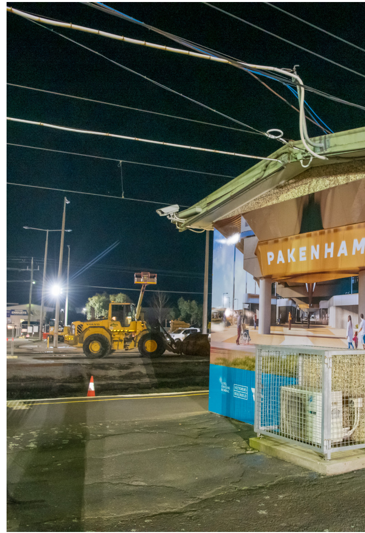
Removing track sidings and preparing the site at Pakenham Station
