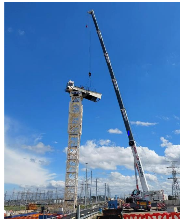
Tower crane installed to construct southern outbound portal
