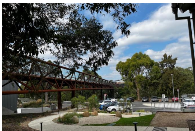
FIGURE 2.11 MORGAN'S WALK UNIVERSITY PEDESTRIAN BRIDGE (SOURCE: SRLA 2022)
