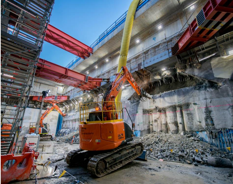
Pile breakout in June
