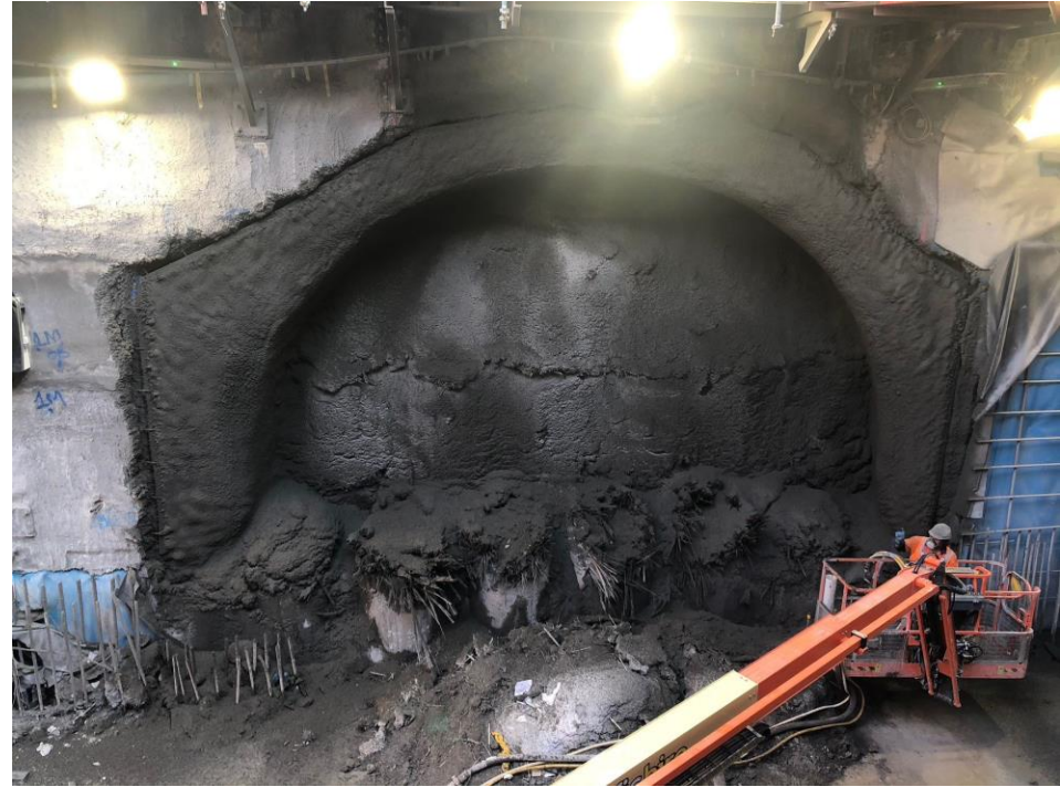
Shotcreting of stub tunnels in July
