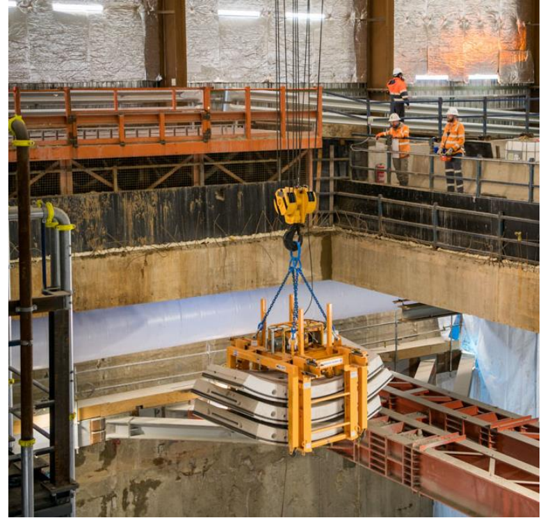
Concrete segments being lowered to the TBM
