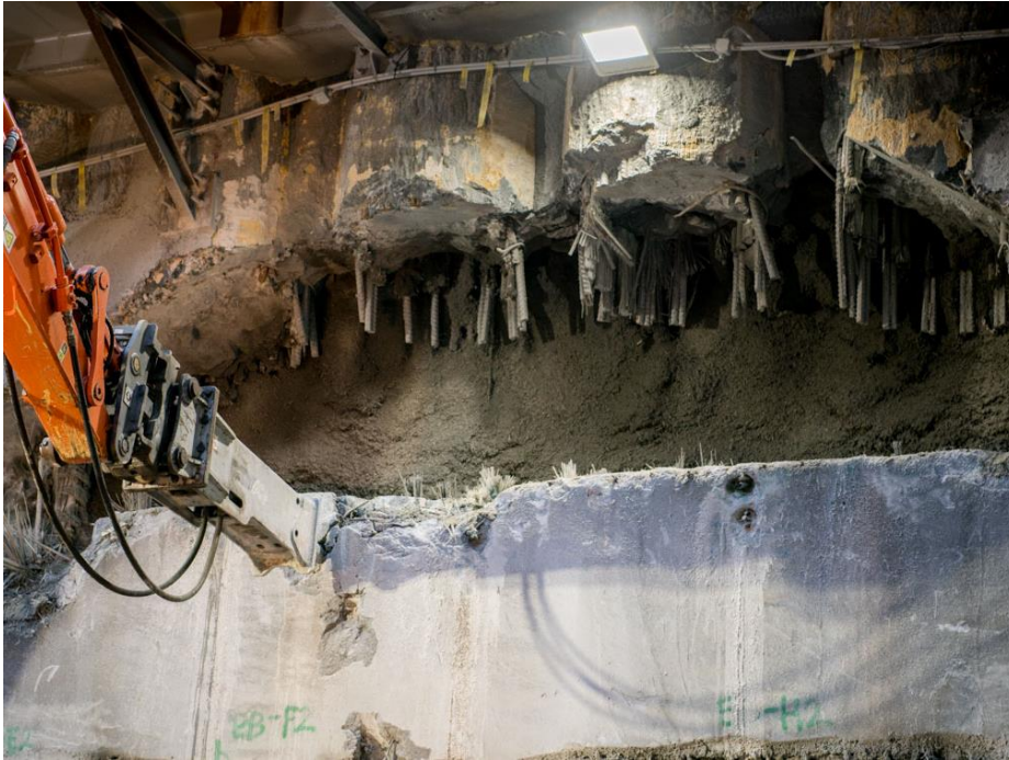
Stub tunnels beginning to take shape
