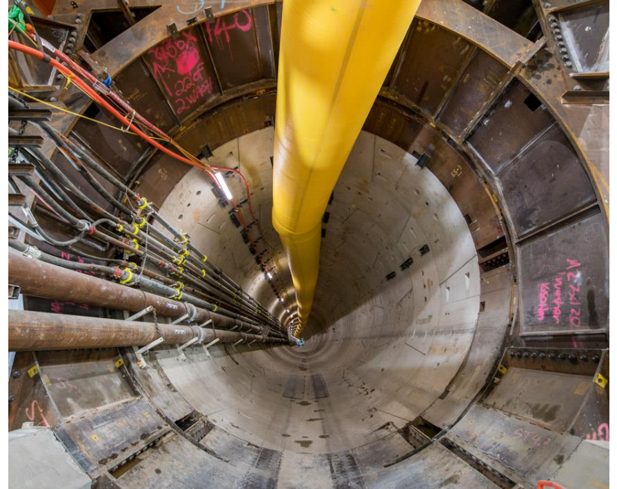
Millie's eastbound tunnel
