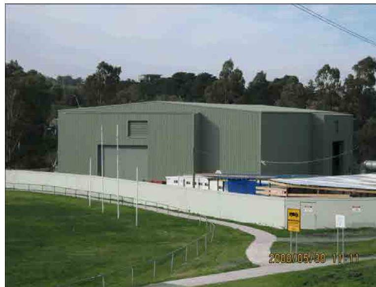
Figure A.43 : Example of acoustic construction shed
