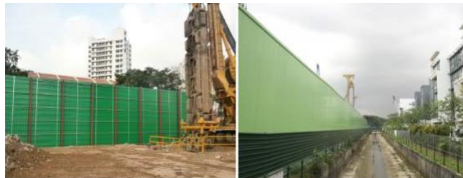
Figure A.42 : Example of noise barriers
