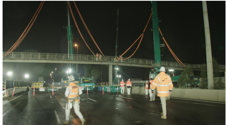
Two cranes at the Rosala Avenue pedestrian overpass
