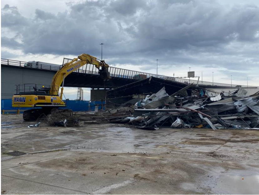
Demolition works at the Socobell site
