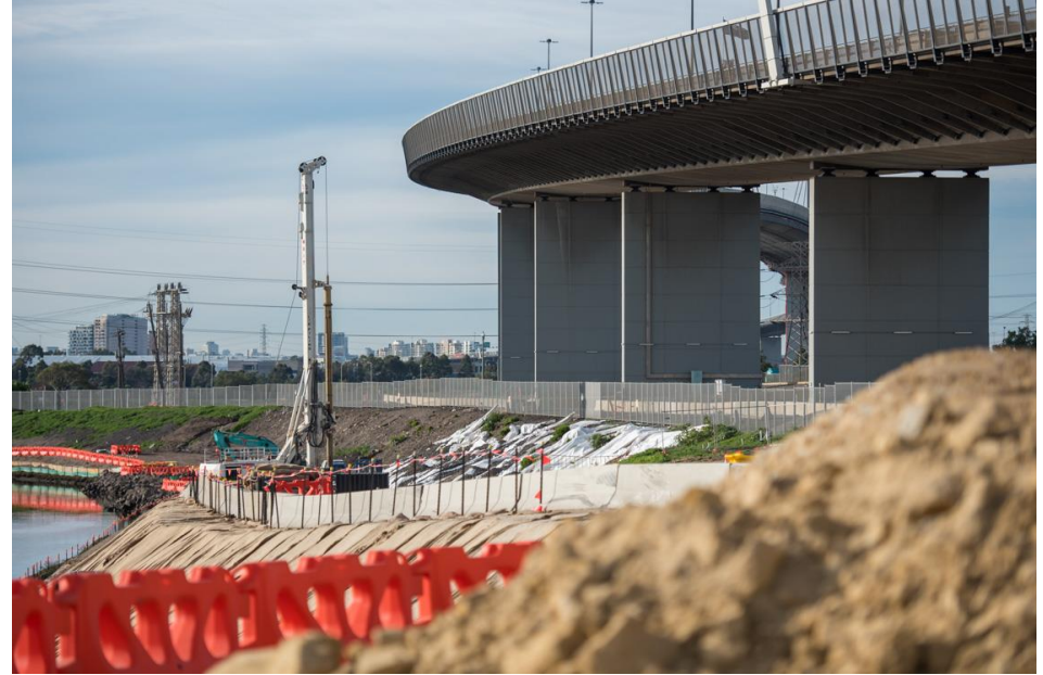
Stony Creek piling
