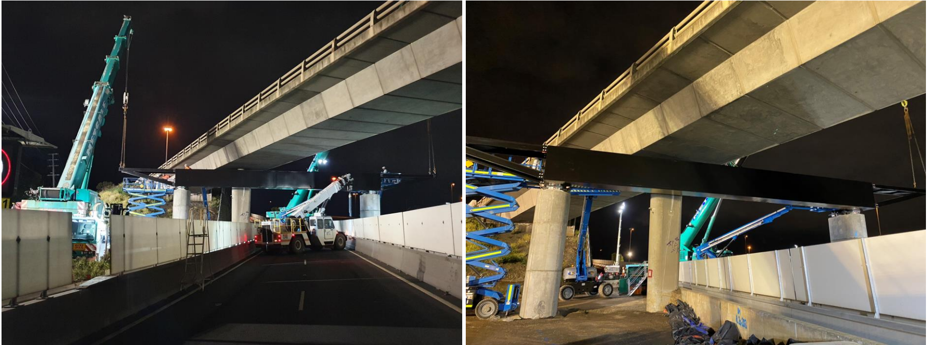
Temporary steel beam supports
