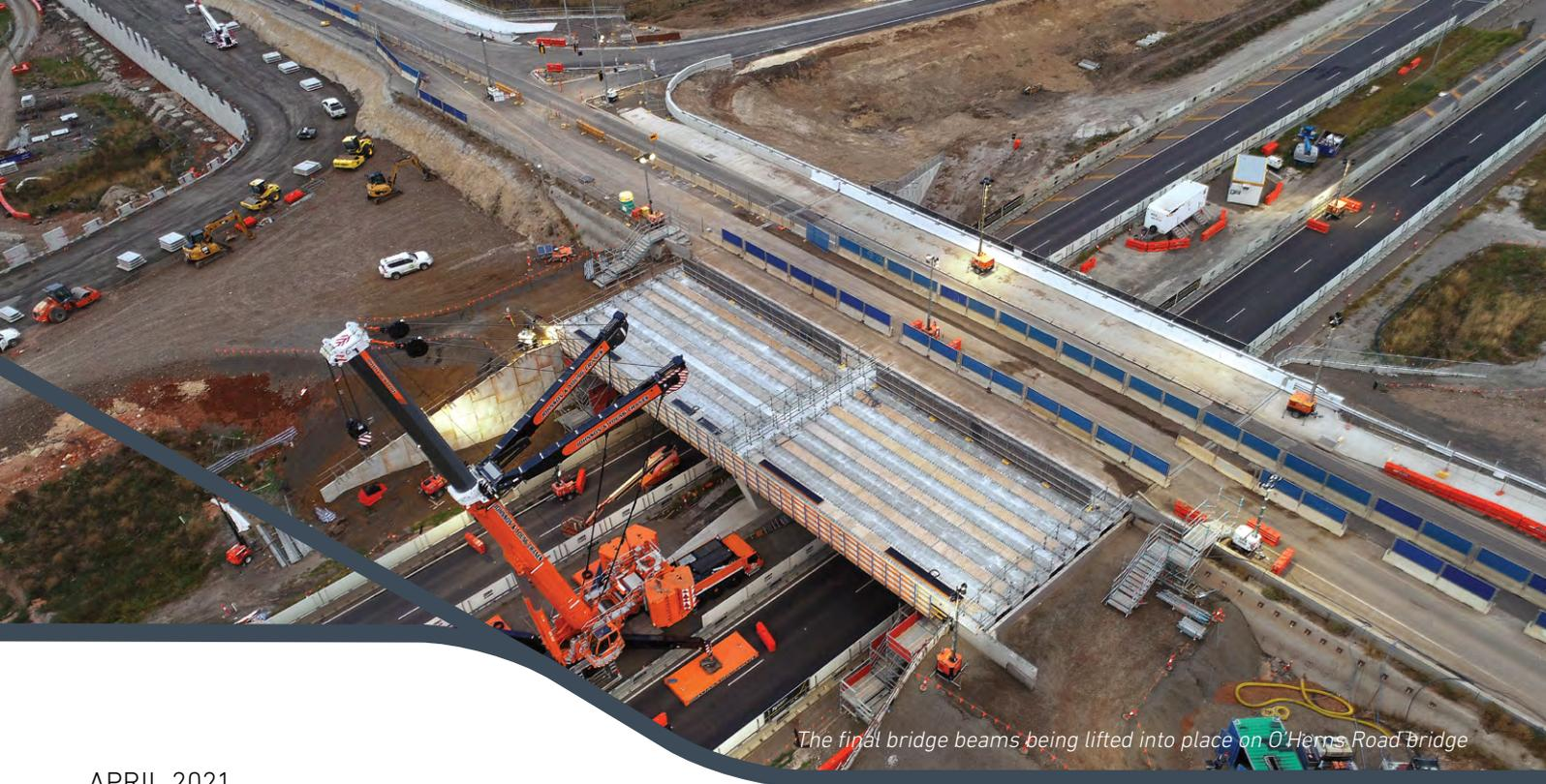
The final bridge beams being lifted into place on O'Herns Road bridge
