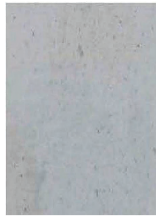
Precast concrete to ancillary building walls - class 2
