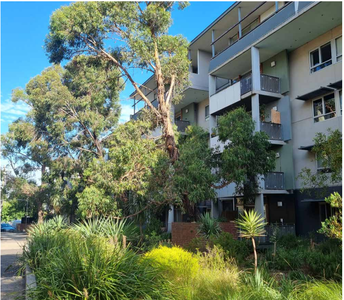
Example of a Water Sensitive Urban Design treatment in Port Phillip
