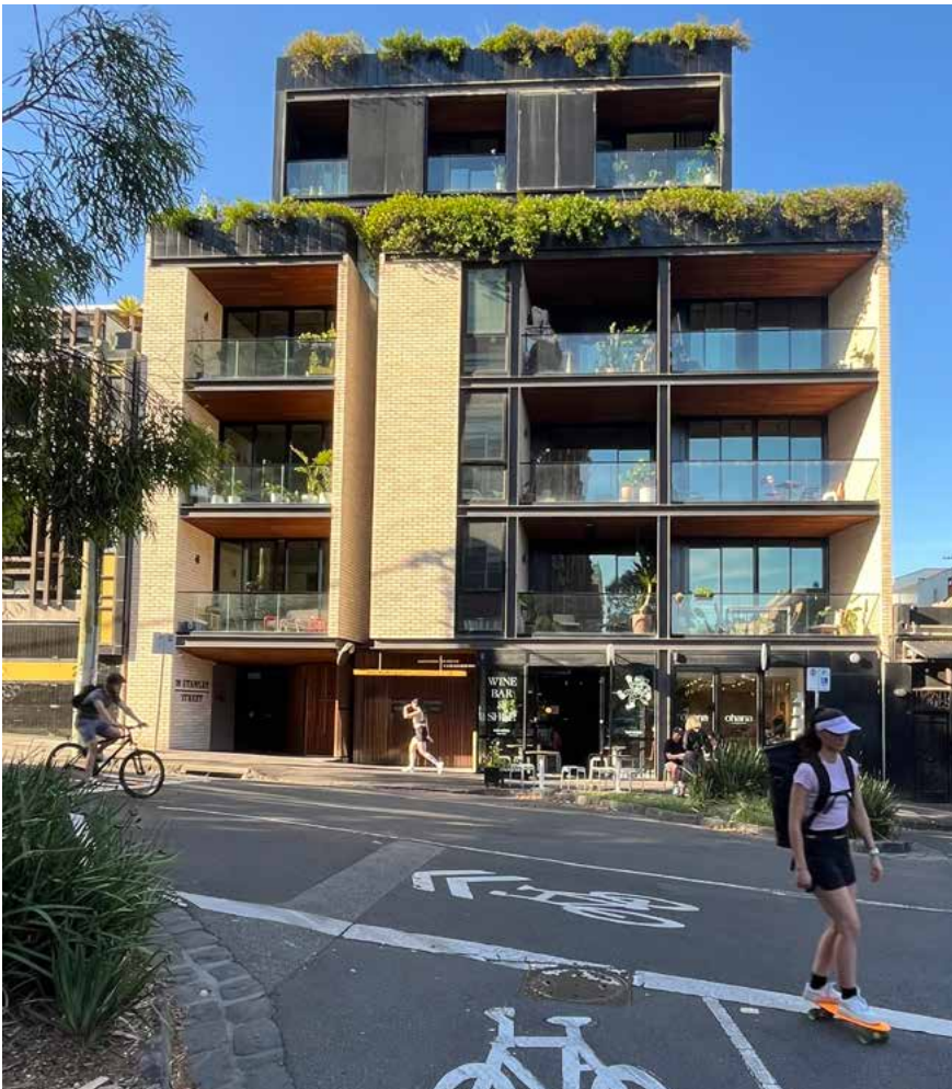
Mid rise apartment development, Stanley Street, West Melbourne
