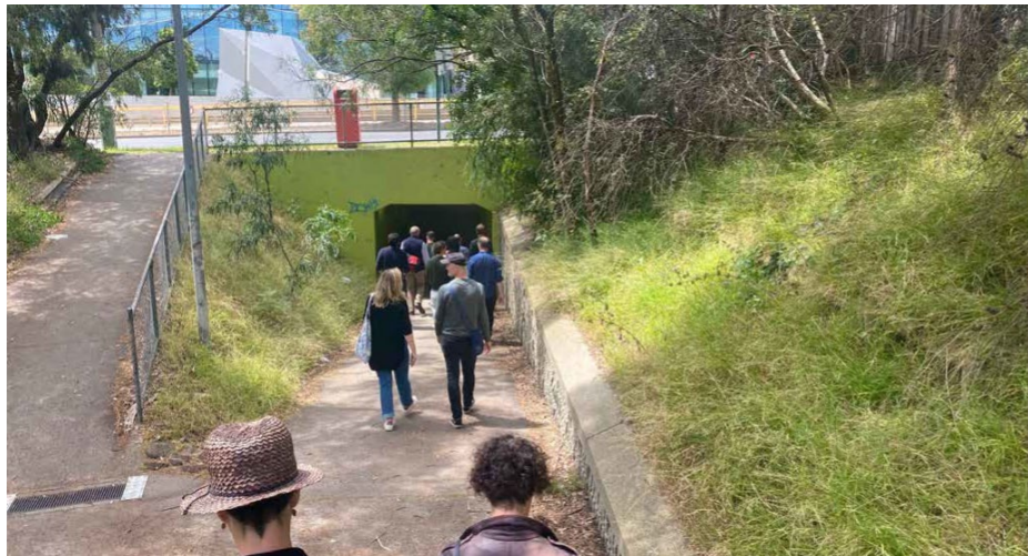
Figure A1.8: Burwood Highway underpass
