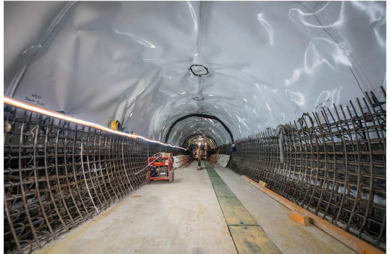
Partially constructed cross passage in Western Precinct, waterproofing membrane and steel fixing
