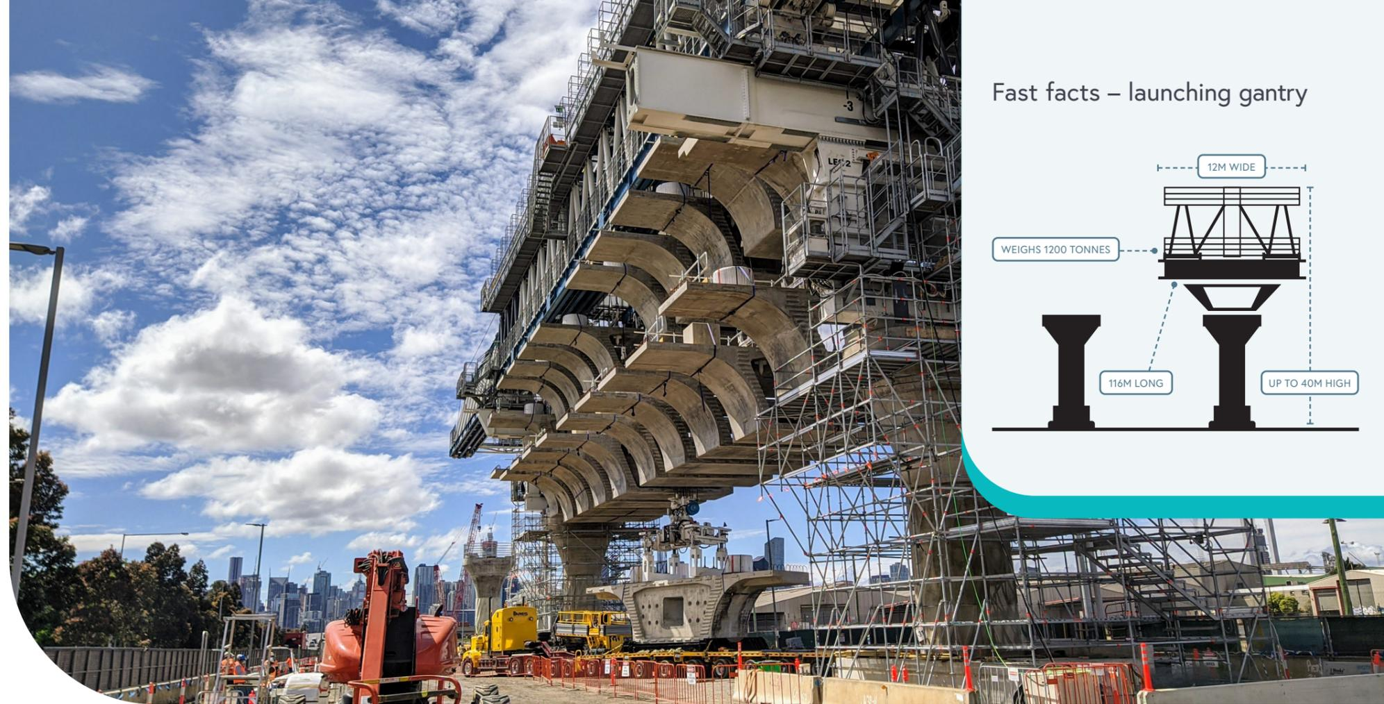
The elevated road builder lifts road segments during testing.
