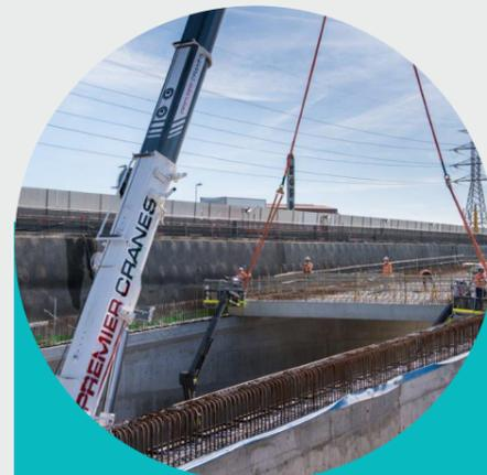
Roof deck installation at the outbound tunnel exit on the West Gate Freeway.
